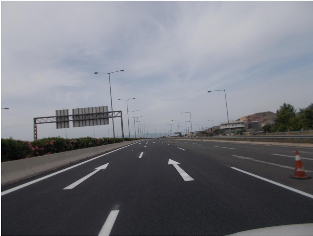
Marking works at k.p. 40+050 to 42+550
