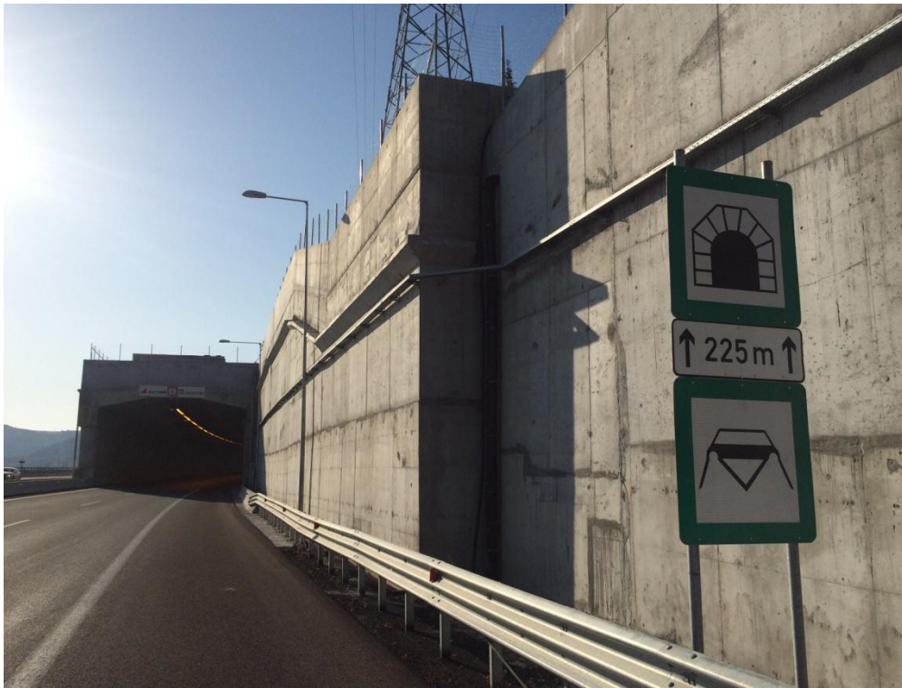
Fencing at side roads
