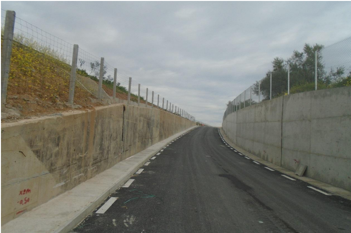
SR003L – Completion of works
