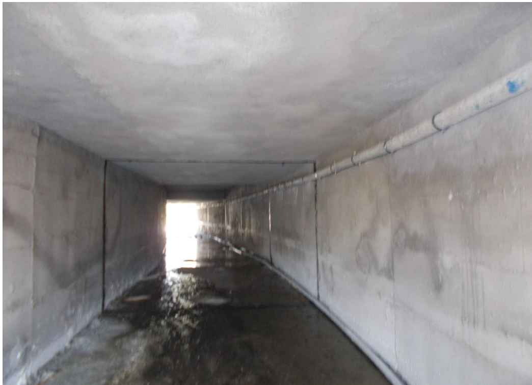
Rehabilitation works at culvert S050
