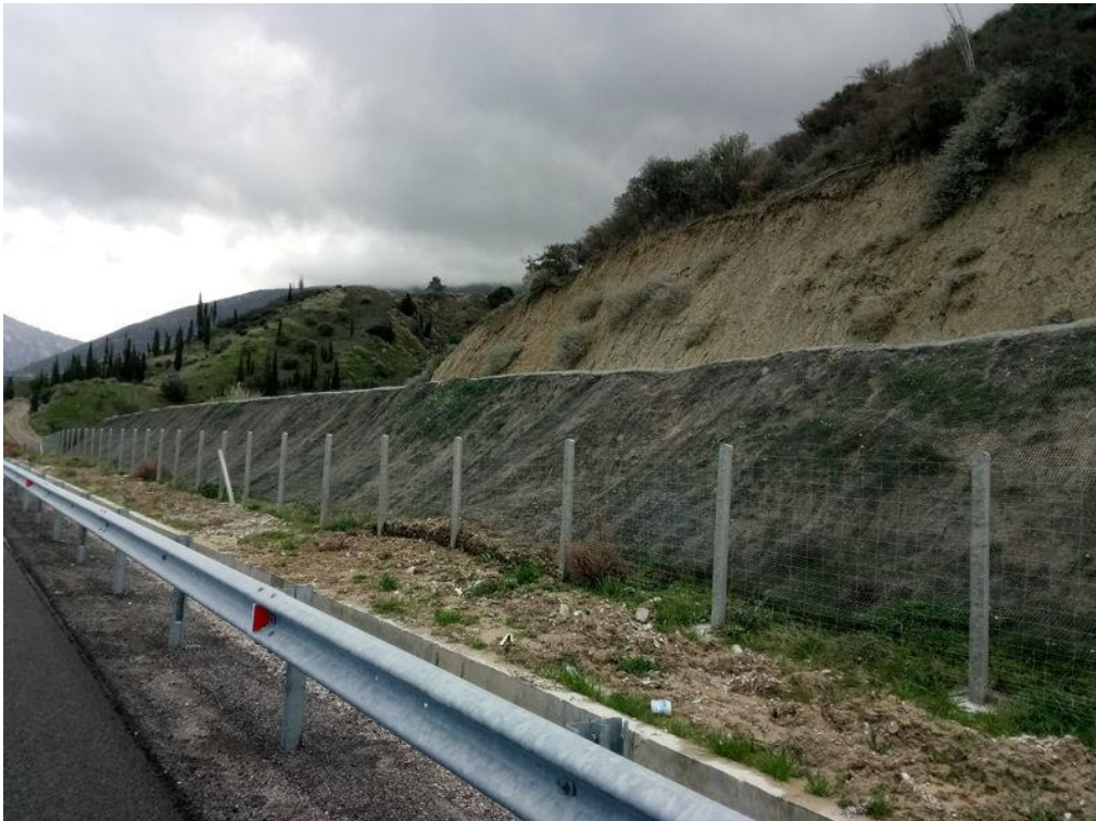
Existing cut 44+170 – 44+230 – Placement of geogrid
