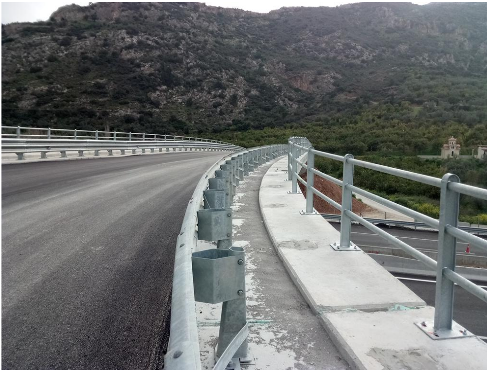
A223 – Replacement of safety barriers and placement of safety guardrails
