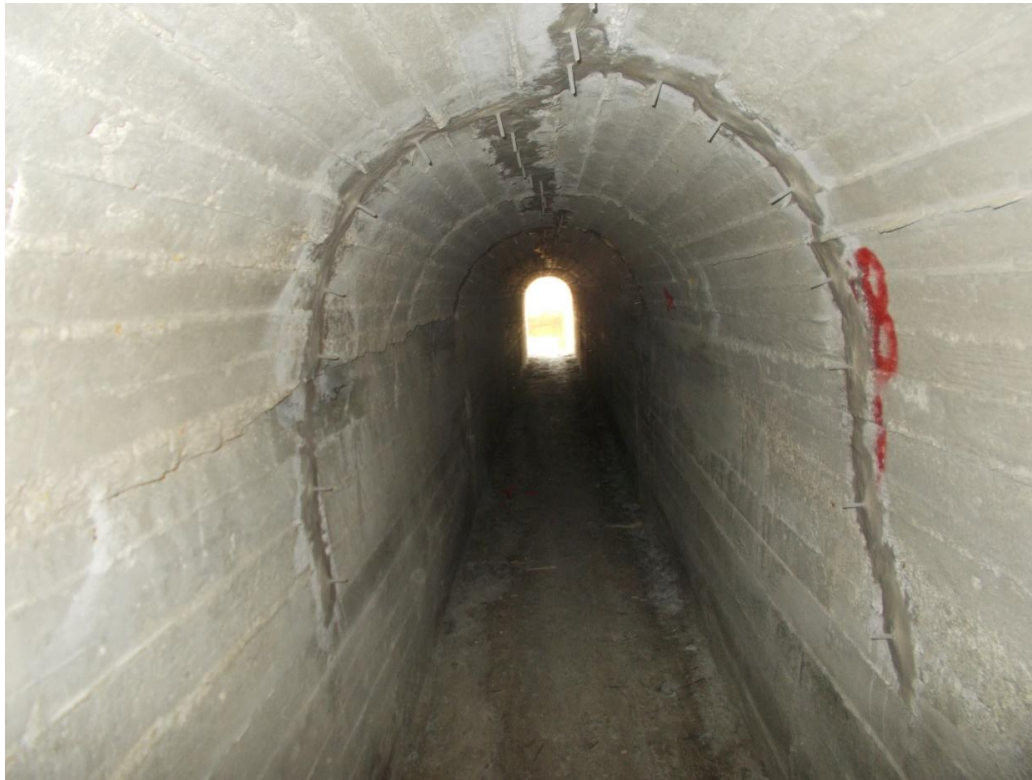
Rehabilitation works at culvert C27
