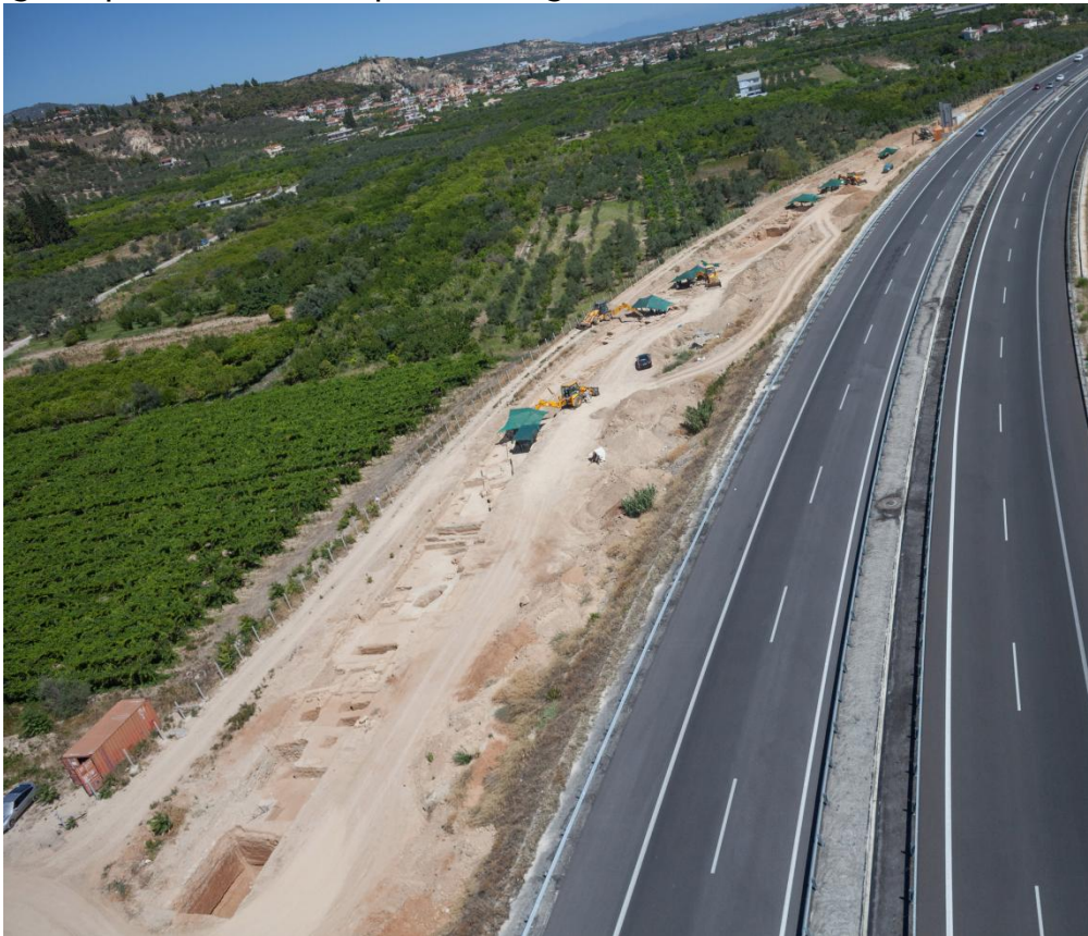
Works in the Archeological site of Asopos - Mouliki (K.P. 17+200, side road)
