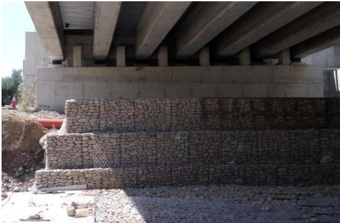
Finikas riverbed arrangement – Construction of M2-A3 gabion baskets
