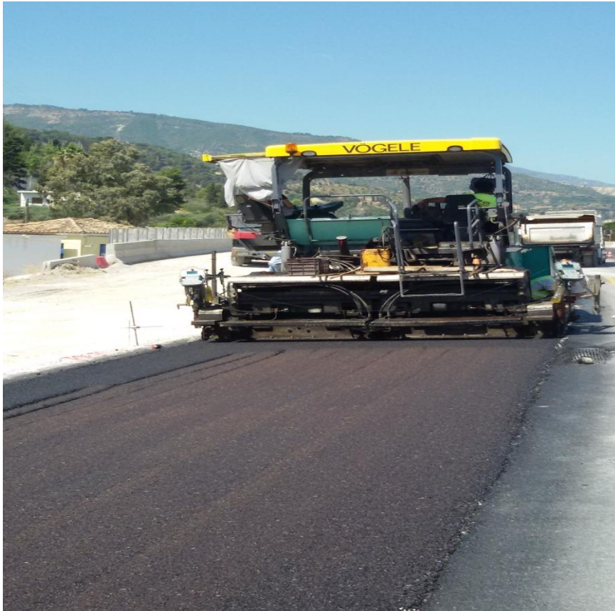
K.p. 52+400-52+810 R.B. - Asphalt works
