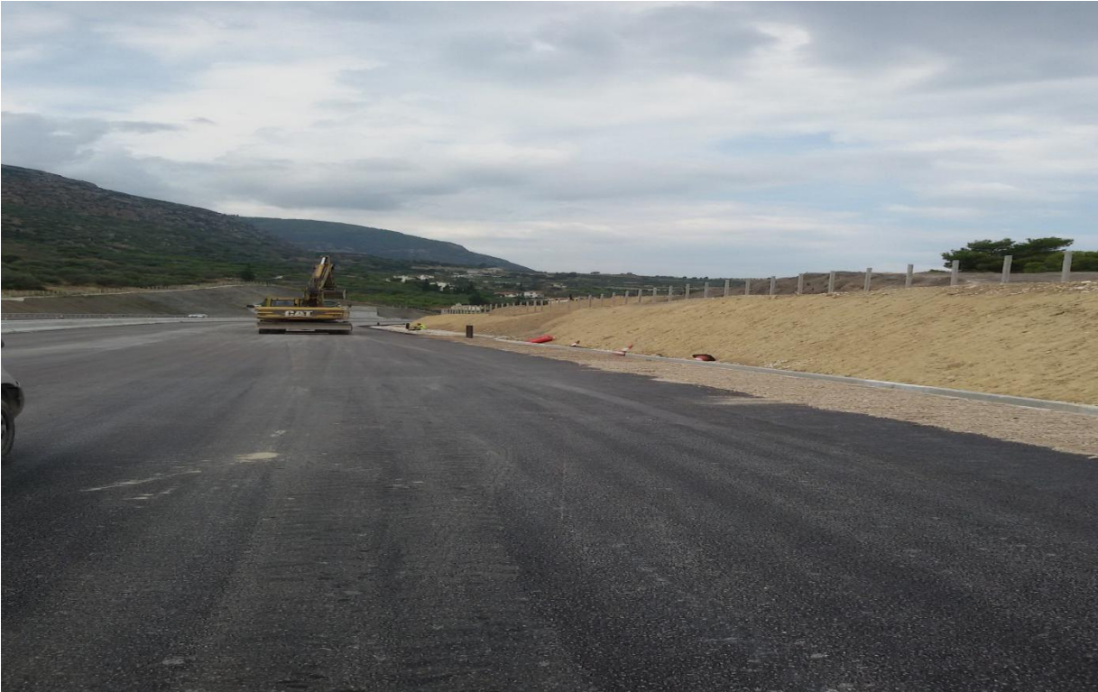
K.p. 33+300-37+000 R.B. - Fencing works
