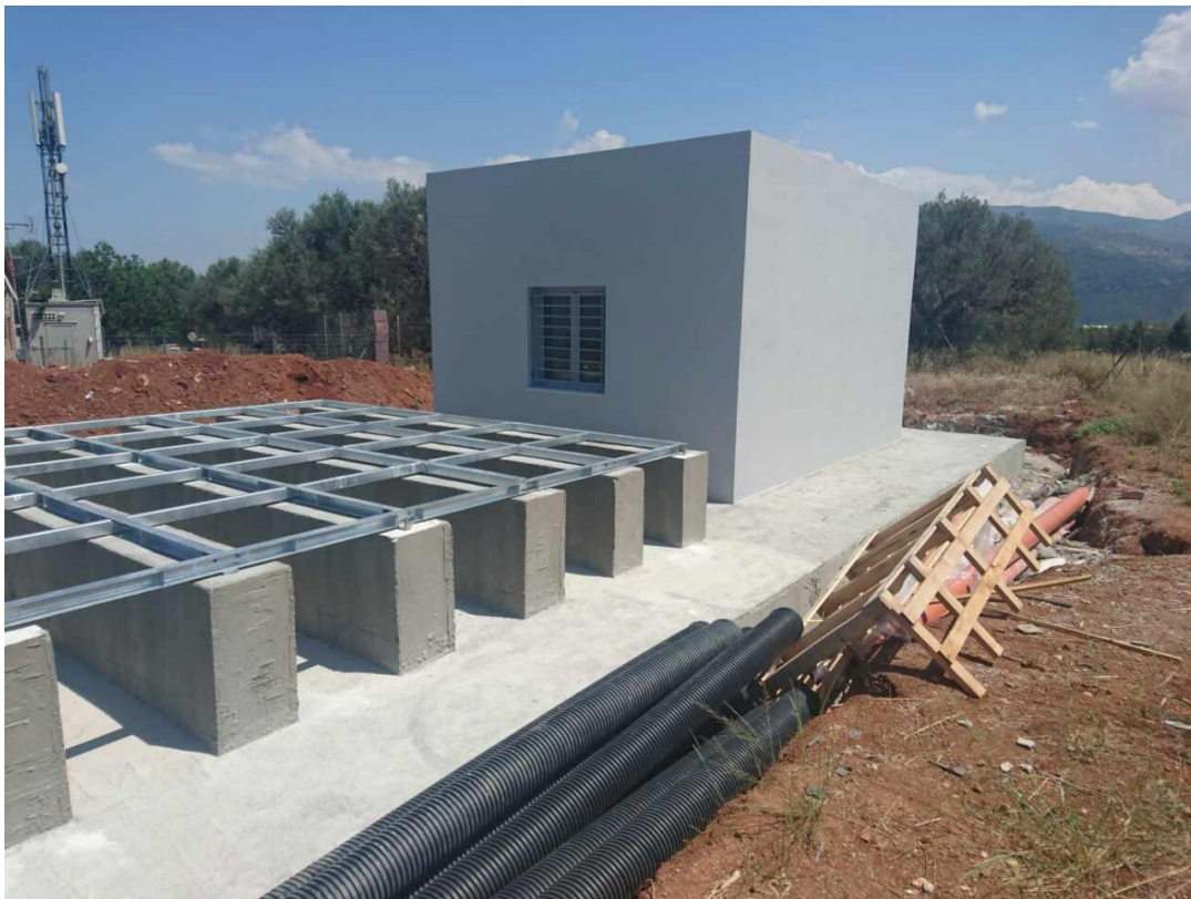
Construction of Pump Station at k.p. 88+040
