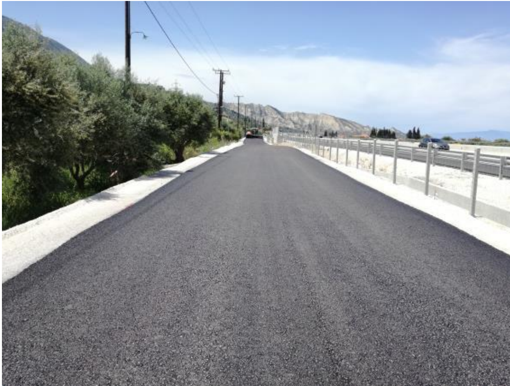
SR033L – Asphalt works of service road
