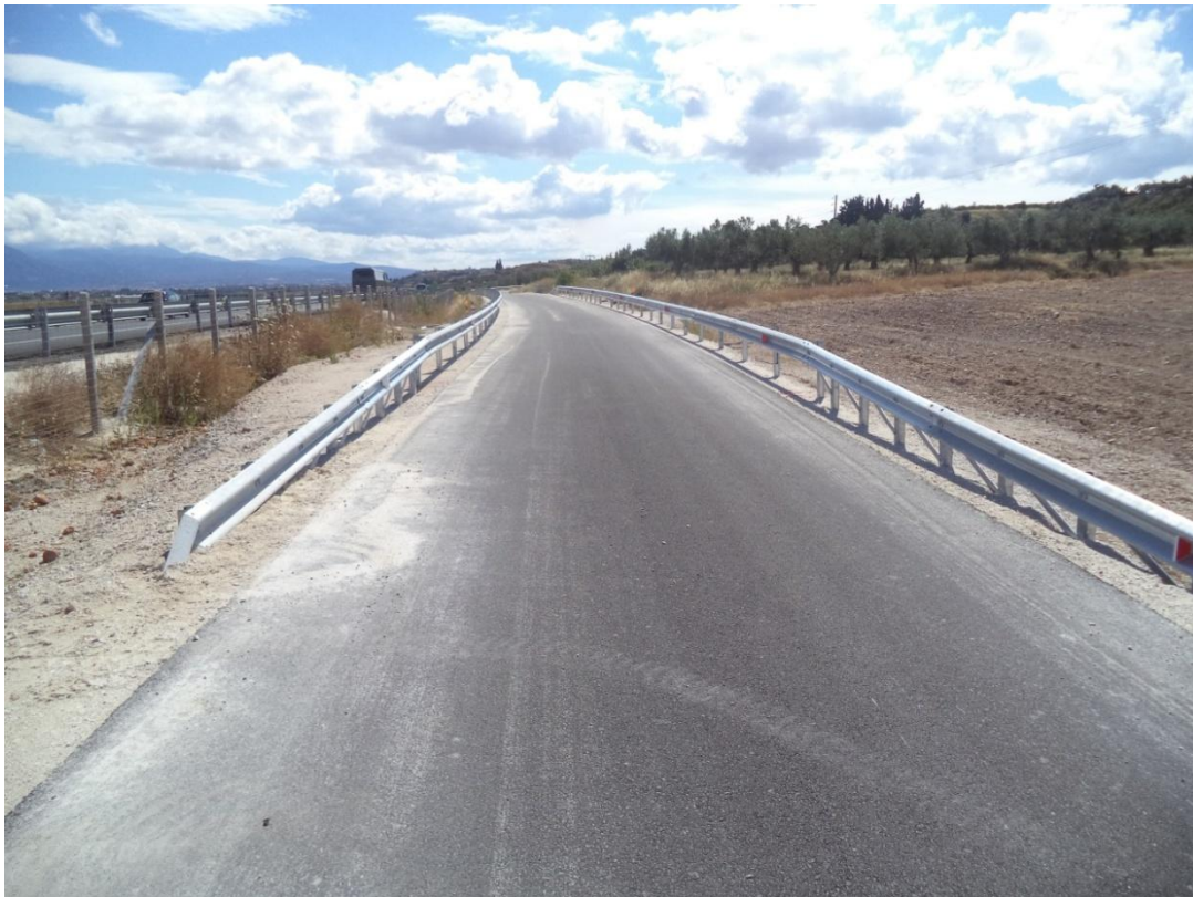
Safety barriers at SR 004L
