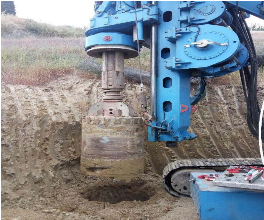
O530 53+174-53+247 L.B.: Drilling of piles
