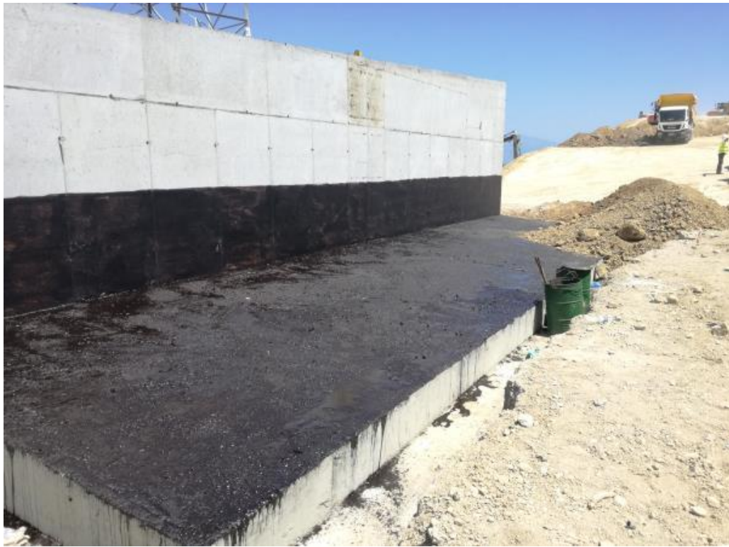
R293 – Construction of retaining wall
