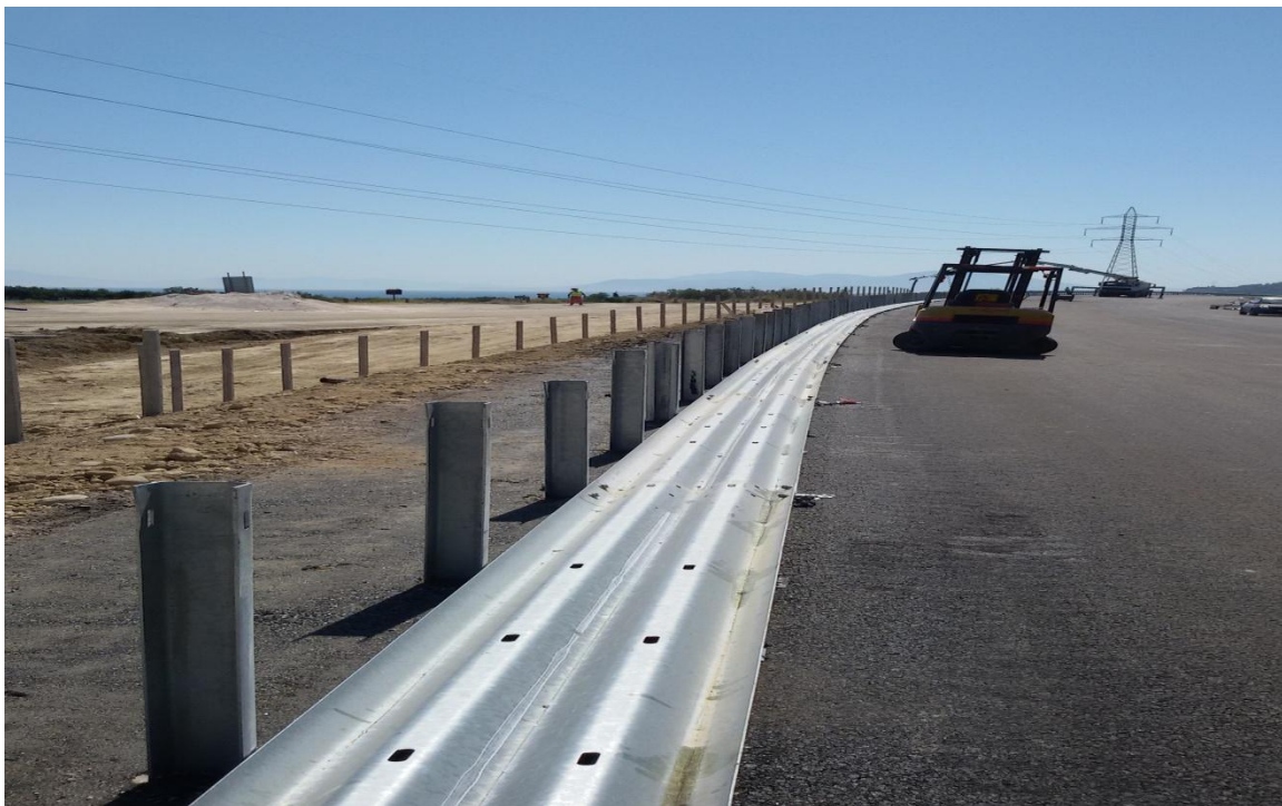
K.p. 33+300-37+000 R.B. - Installation of steel safety barriers
