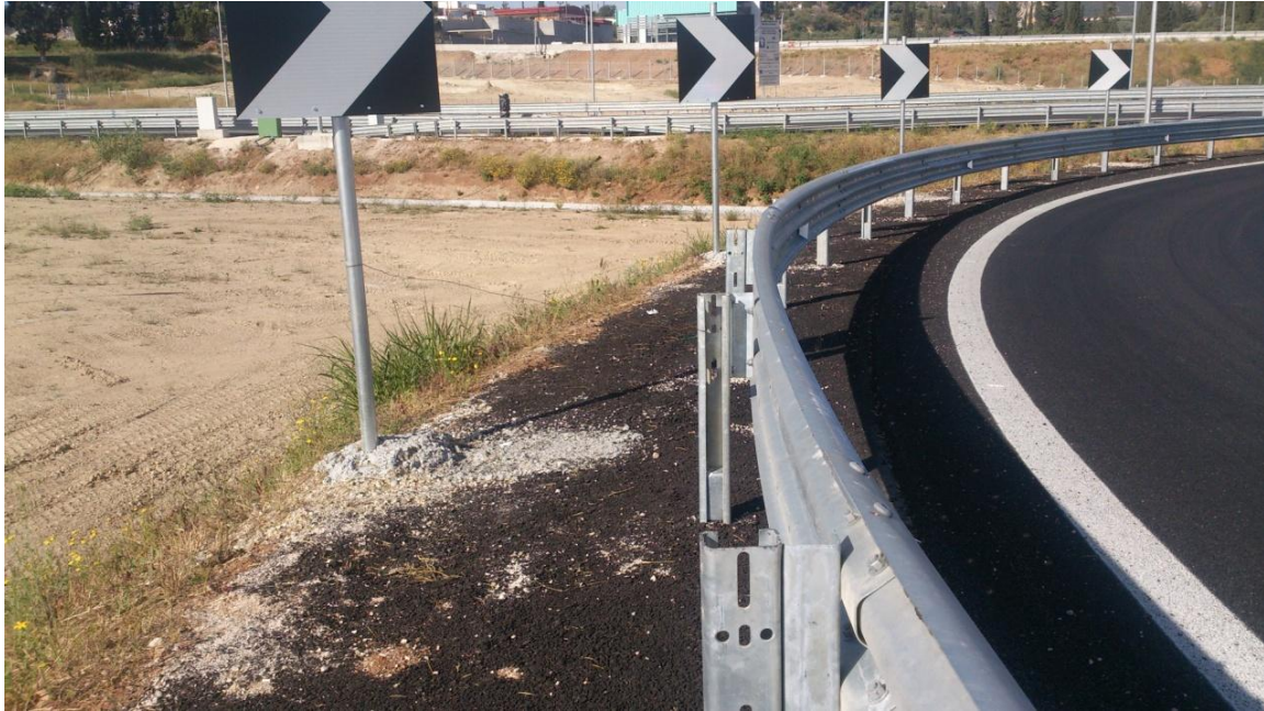
Installation of side signs
