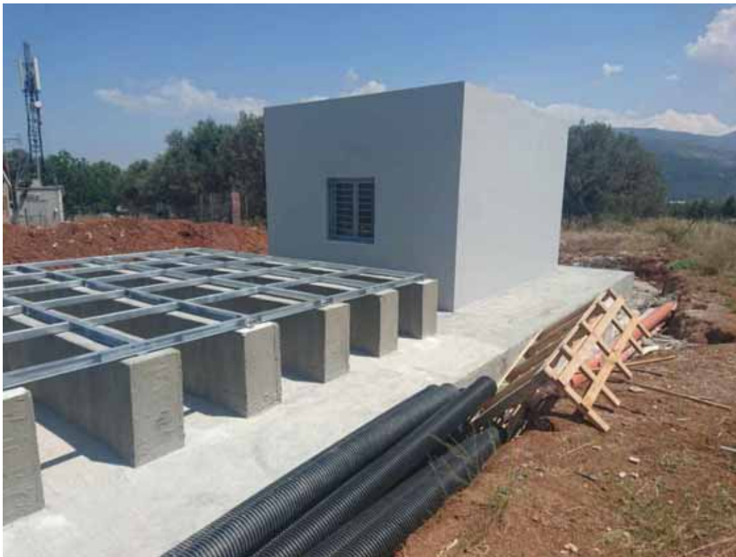
Construction of Pump Station at k.p. 88+040
