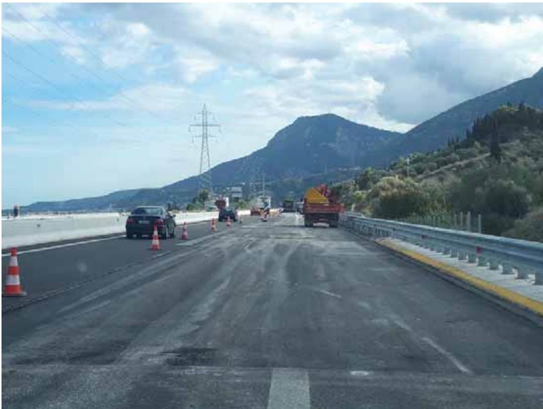
Rehabilitation of asphalt defects at k.p. 45+221
