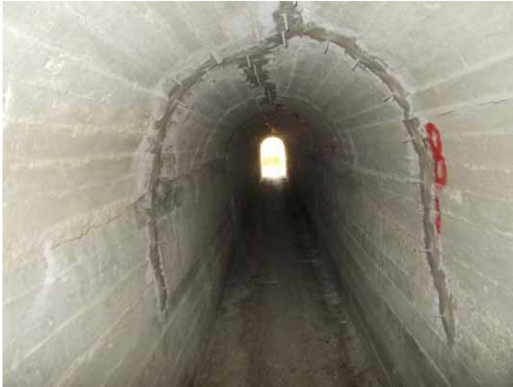
Rehabilitation works at culvert C27
