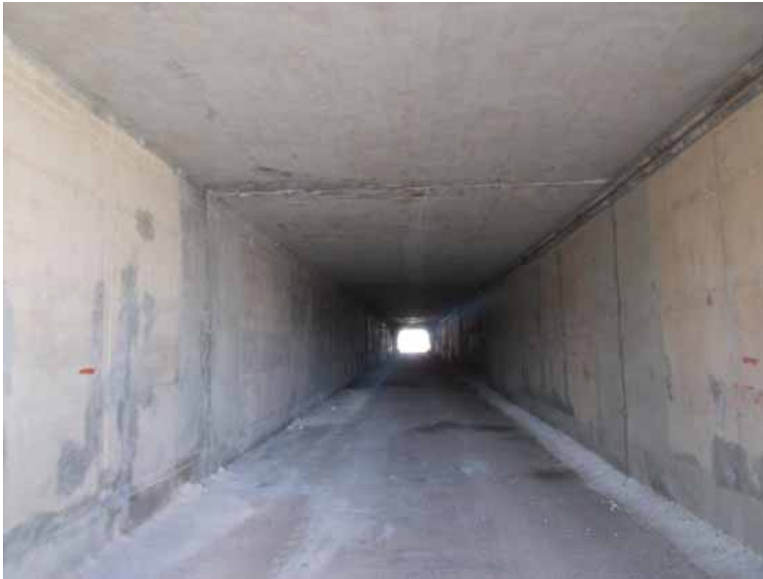
Rehabilitation works at culvert S46 (ΓΕ 1-15)
