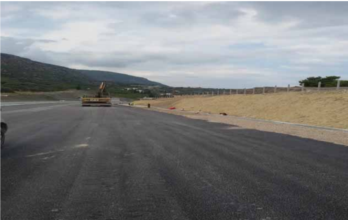
K.p. 33+300-37+000 R.B. - Fencing works
