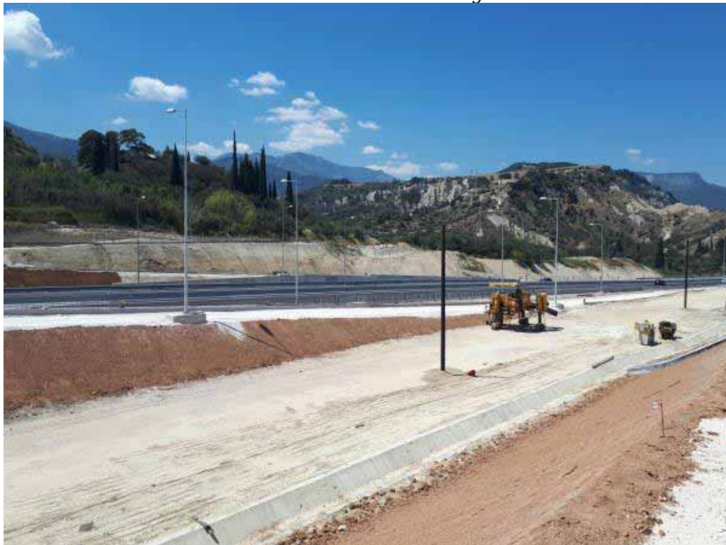
Interchange of Lykoporia – Installation of cables, bases and lighting poles
