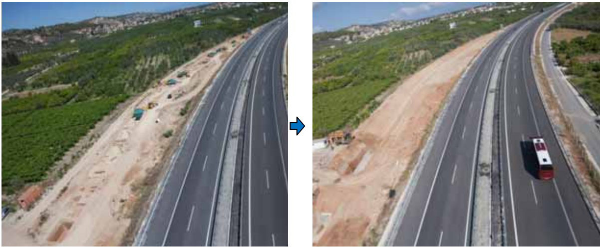
Works in the Archeological site of Asopos - Mouliki (K.P. 17+200, side road)
