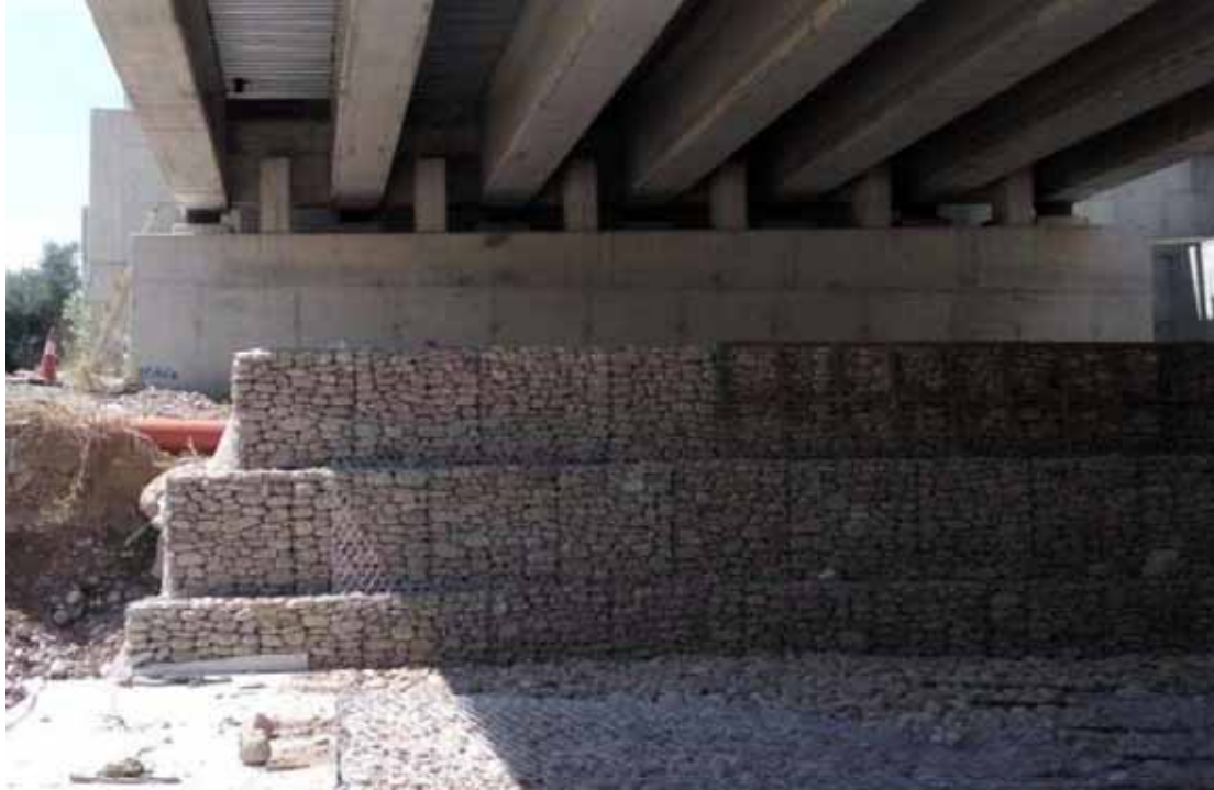
Finikas riverbed arrangement – Construction of M2-A3 gabion baskets
