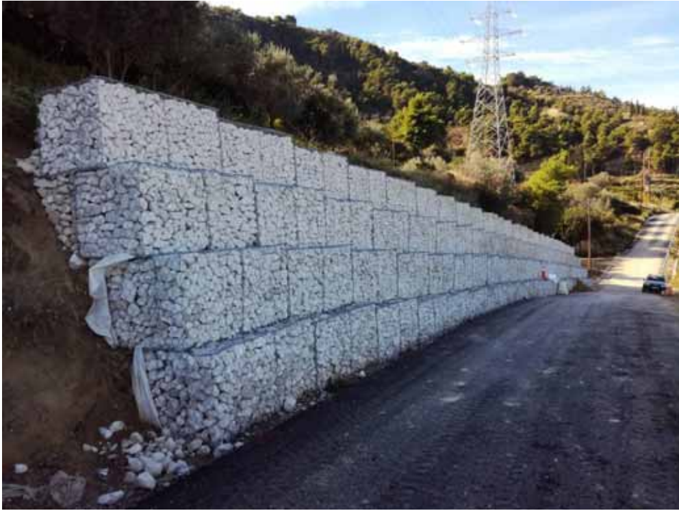
G285 – Gabion wall construction
