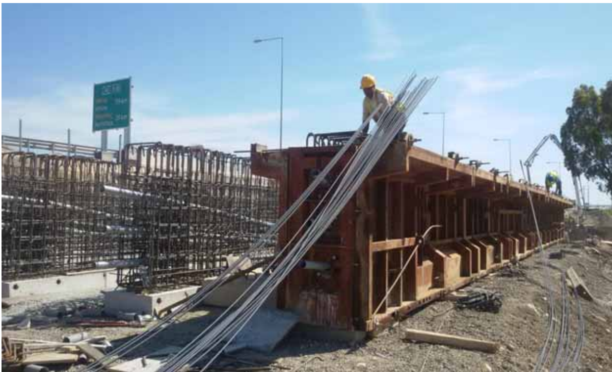
B211 (SR KP 32+763) - Construction of precast beams
