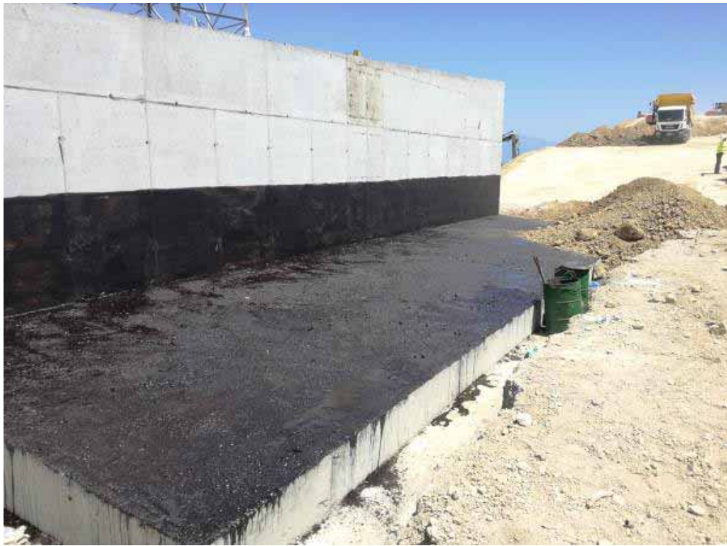
R293 – Construction of retaining wall
