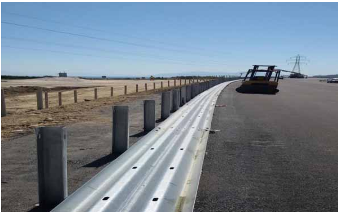
K.p. 33+300-37+000 R.B. - Installation of steel safety barriers
