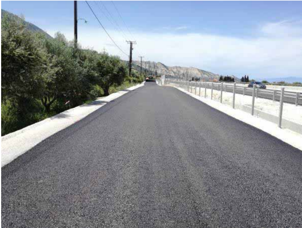
SR033L – Asphalt works of service road
