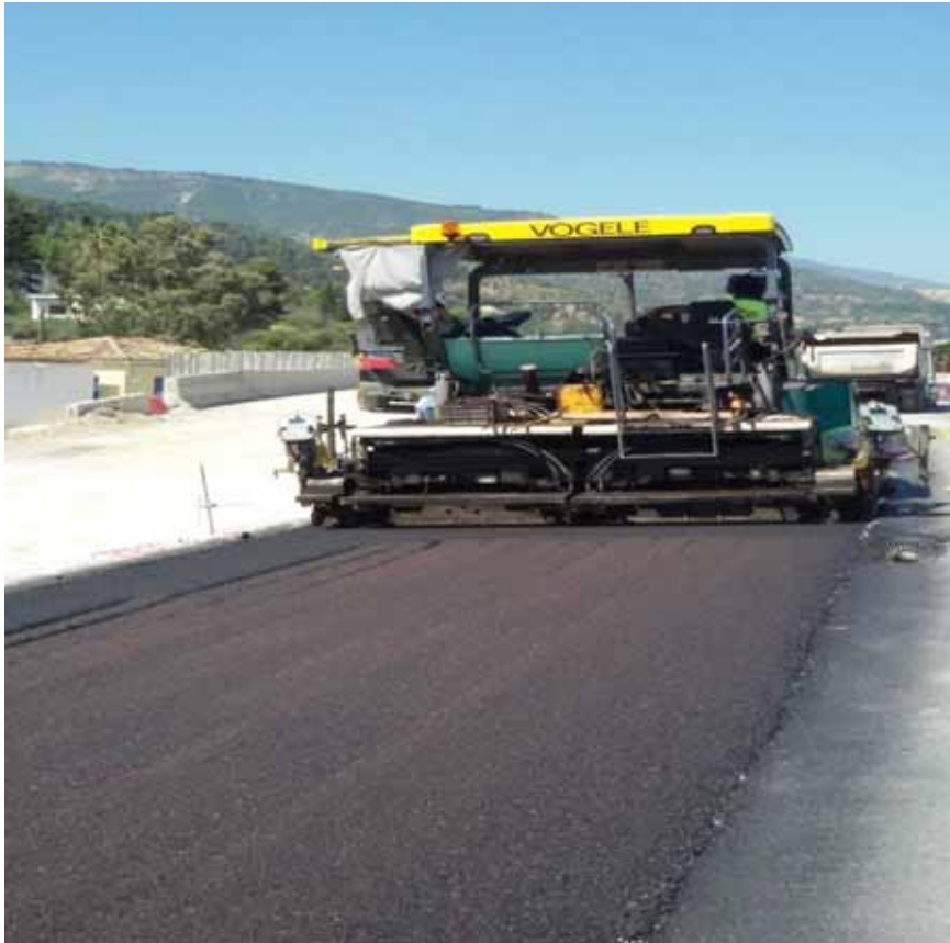
K.p. 52+400-52+810 R.B. - Asphalt works
