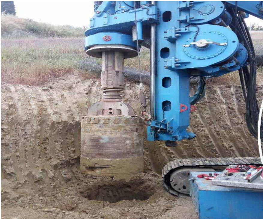
O530 53+174-53+247 L.B...: Drilling of piles
