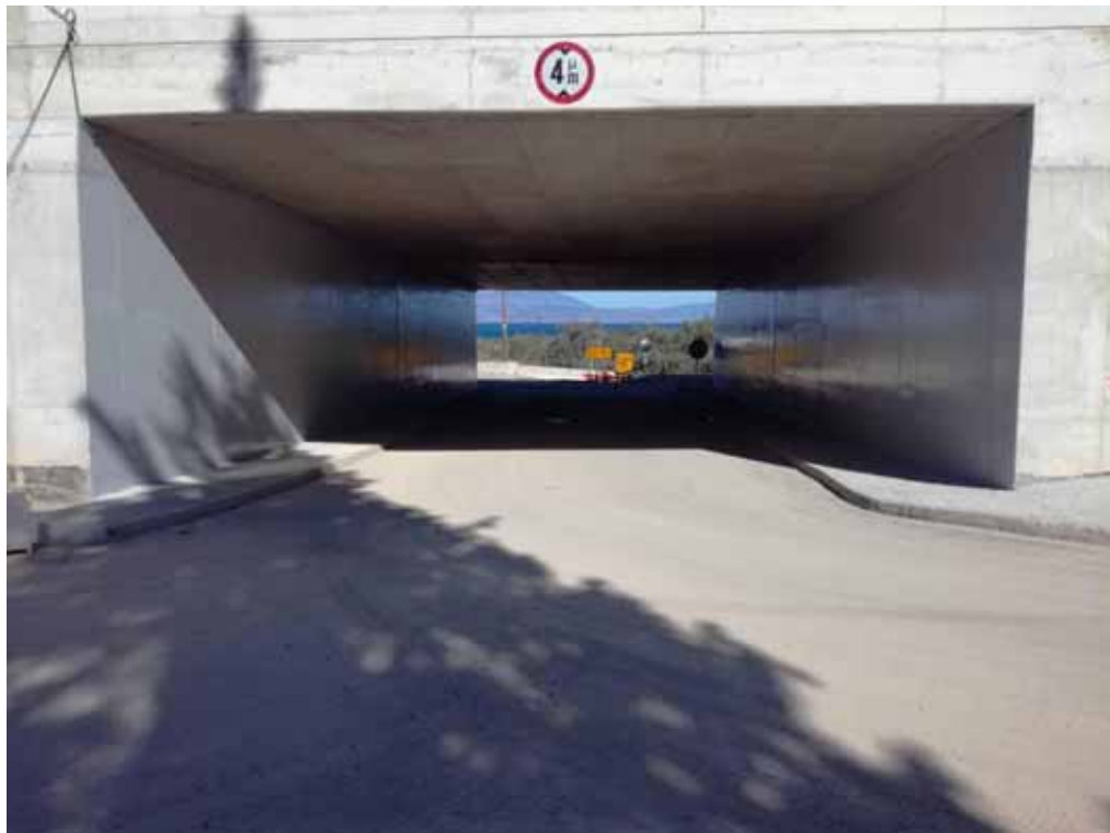
K238 – Antigrffiti coating implementation
