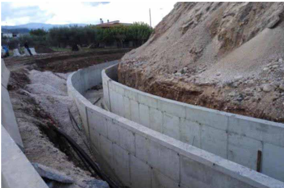
Construction of drainage ditches at Aigio MSS
