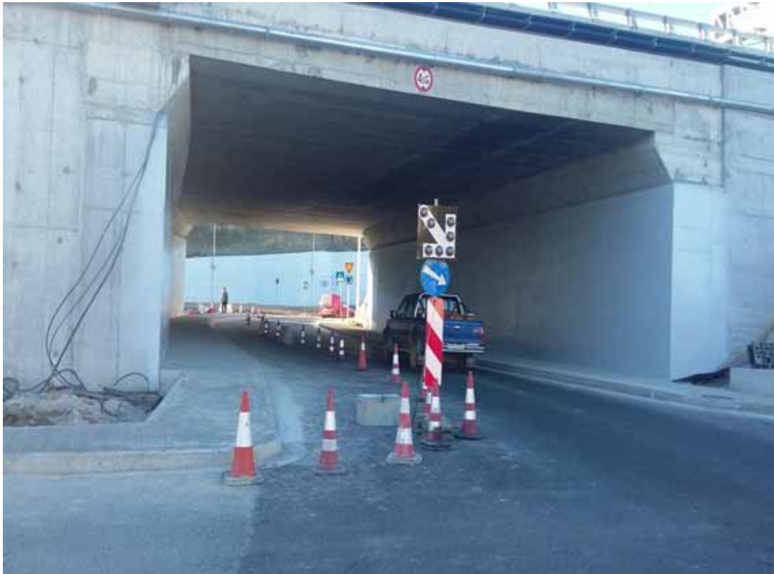
K217 – Sidewalk construction
