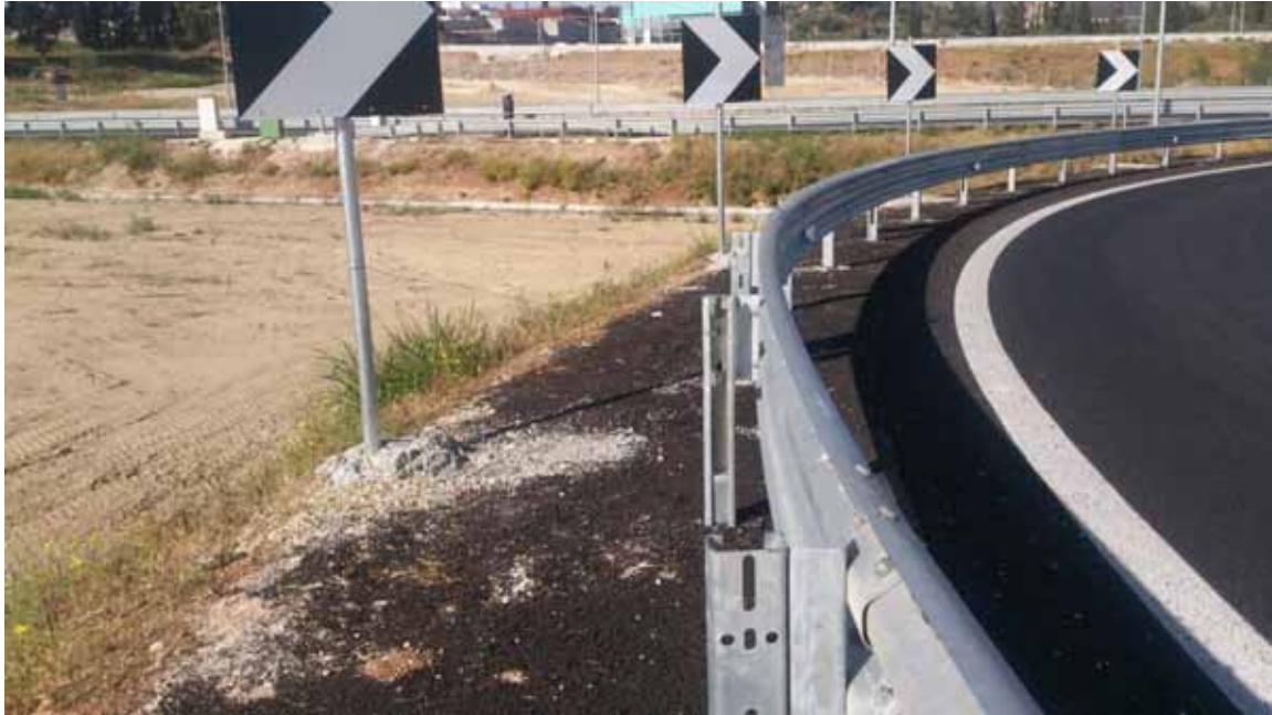
Installation of side signs
