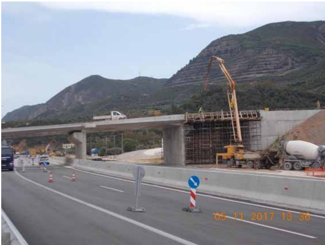
Overpass A344 at Arachovitika I/C
