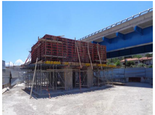
B322 – Construction of M3-M4
