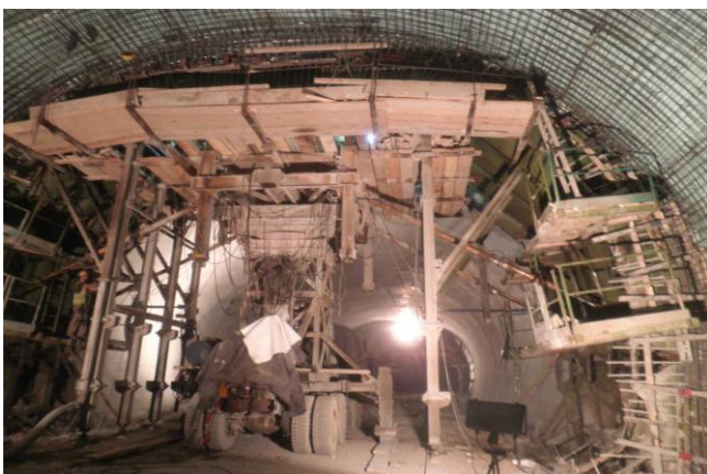
Tunnel Platanos/ East Portal – Construction of final lining
