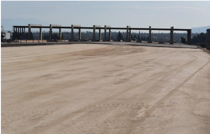
Pavement works at Nikoleika Toll Station k.p. 78+050 to 78+250
