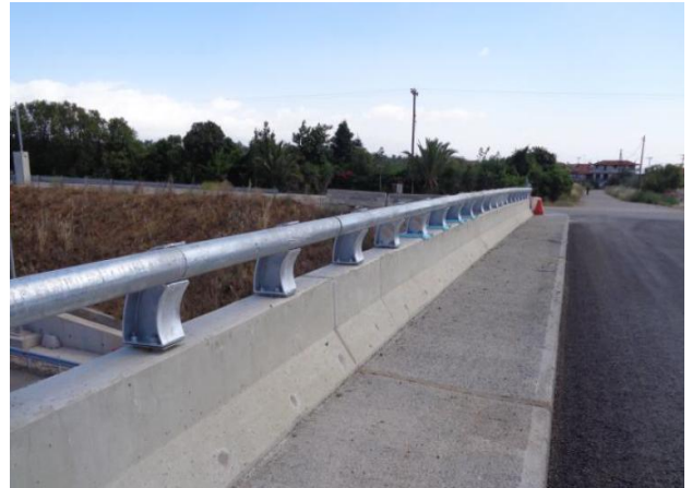
A293 – Installation of safety guardrails
