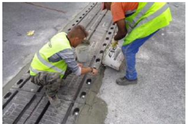
B278– Installation of expansion joints
