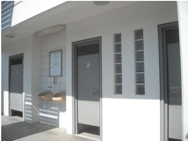
WC Buildings – Finishing works
