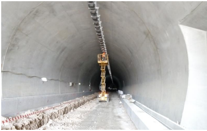
Tunnel Platanos/North Bore – Installation of E/M infrastructures
