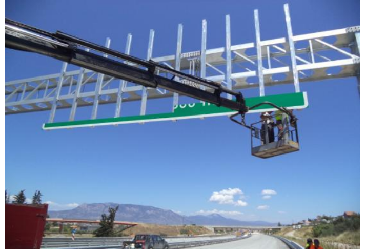
Installation of Information sign
