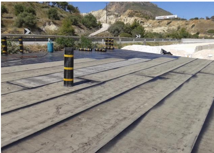
Underpass K221 – Deck waterproofing
