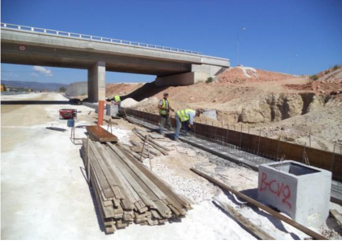
Construction of drainage at k.p. 7+900 to 9+500
