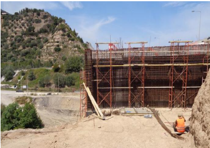
B269 – Construction of left backwall
