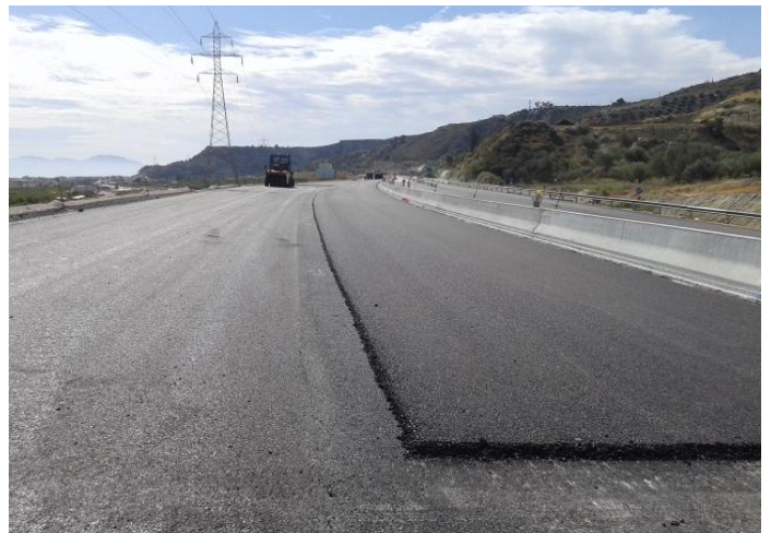
Asphalt works/AS20 at k.p. 34+350 to 34+600
