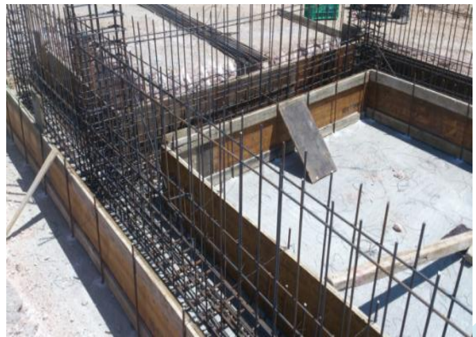
Construction of Customer Service Center
