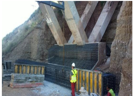
A296 – Strengthening footing and constructing pilewall at M1
