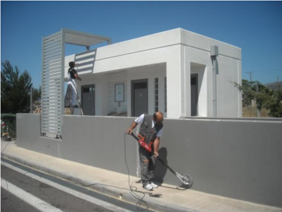
W/C building at N. Peramos parking area – Painting works
