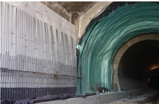
Final lining – Waterproofing of Vault (West Portal/North bore)
