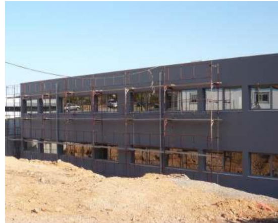
Painting works at MOMC Unit 1 – North part
