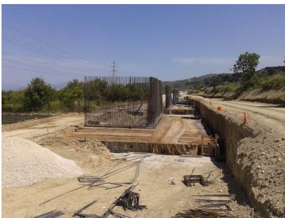
Construction of retaining structure R274
