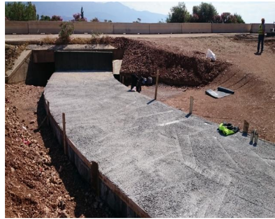
Construction of L518
