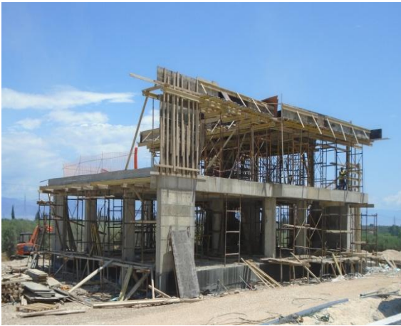
Construction of Toll Service Building at Nikoleika
