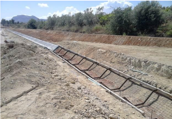
Construction of EDL011L109
