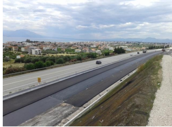
Asphalt works at k.p. 21+300 – 22+760
