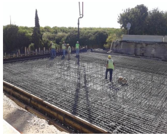
Bridge B204 – Pouring of top slab
