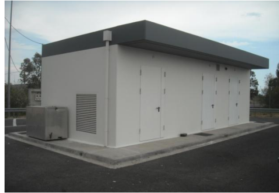
M Building at Pachi Toll Station – Painting works
