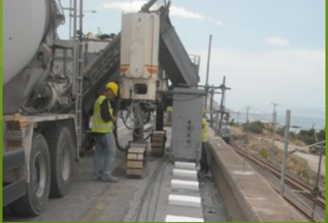
Concrete works with the slip forming machine
