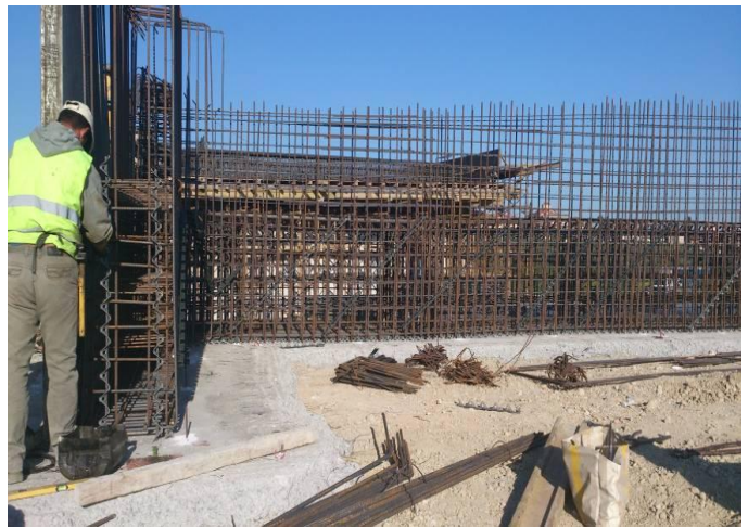
Construction of Abutment A0, A137
