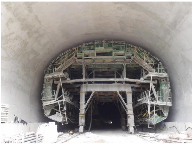
Cut & Cover T007 West: segment 2
