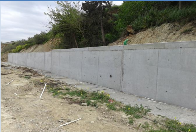
Retaining Structure G247
