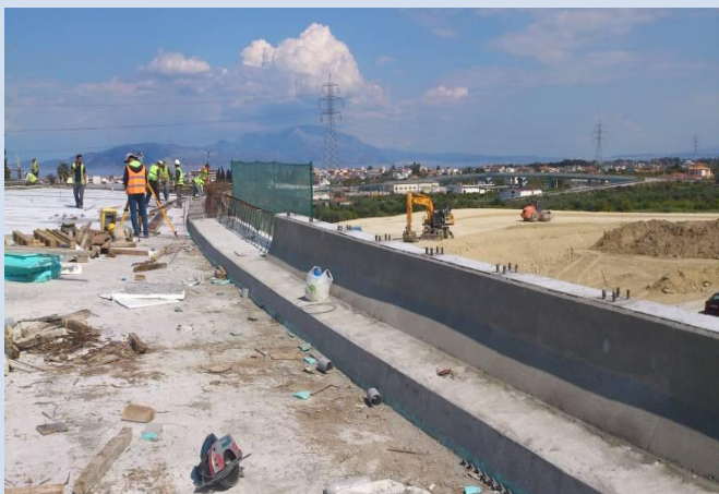
Construction of top slab, A137
