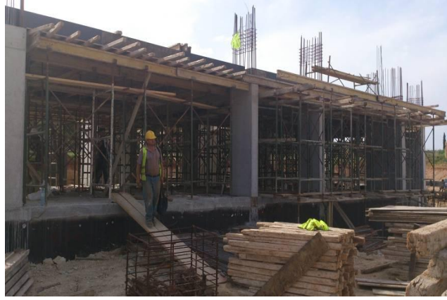
Construction of TAB, k.p. 18+800
