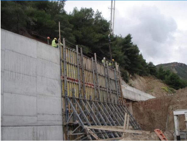
G309 Walls concrete
