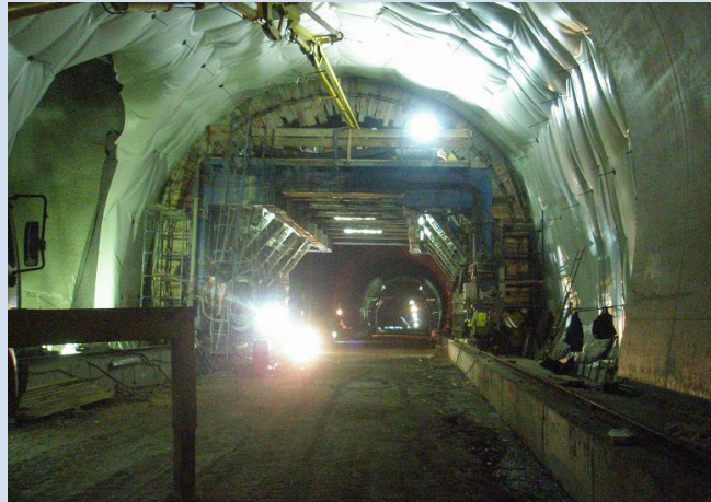
Mavra Litharia Final Lining-Concrete works
