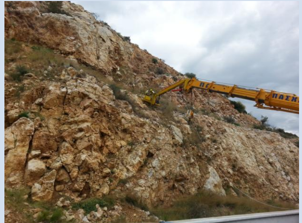
Loose rock removal
