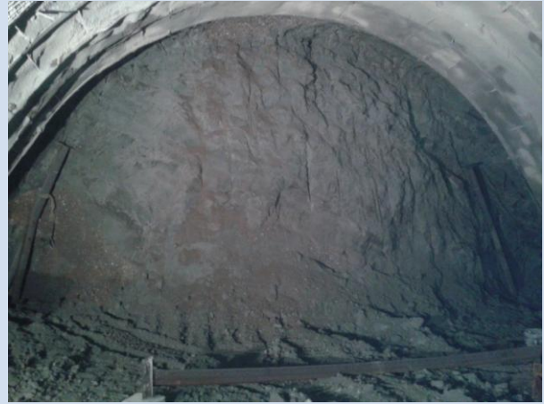
North Bore - A' Excavation Phase
