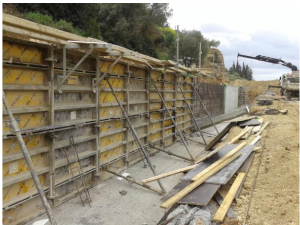
Retaining Wall G246: construction of foundations & wall's stems
