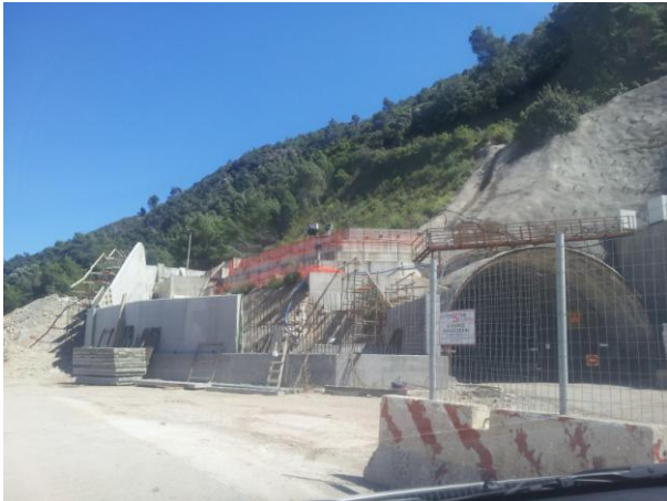
T26_NW retaining walls
