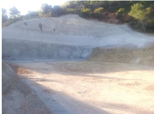
T25_west portal cover & cut open excavation
