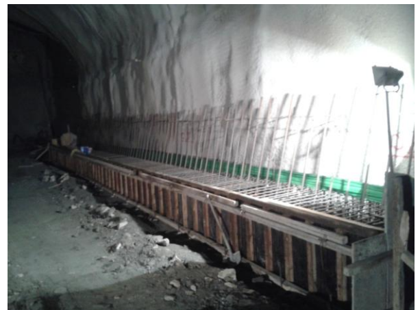
Implementation of final lining - (Footing) Cross Passage 2
