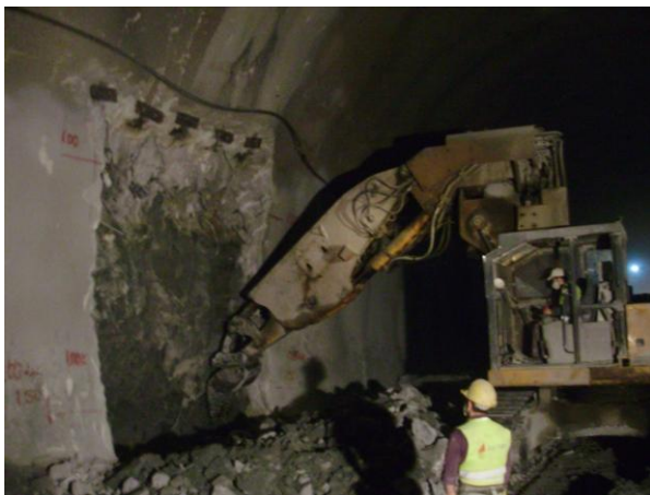
South Bore - B' & C' Excavation Phase
