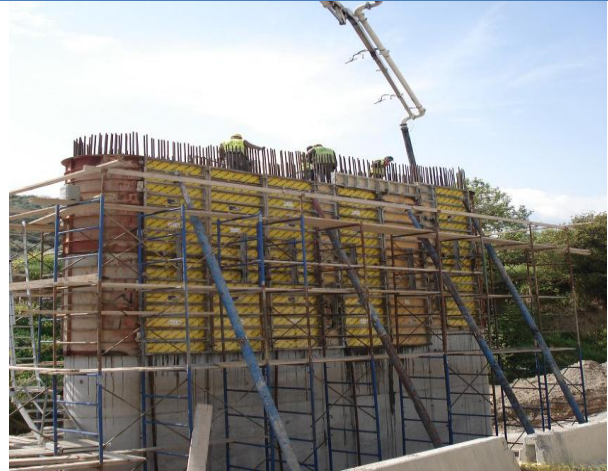
G309 Walls concrete
