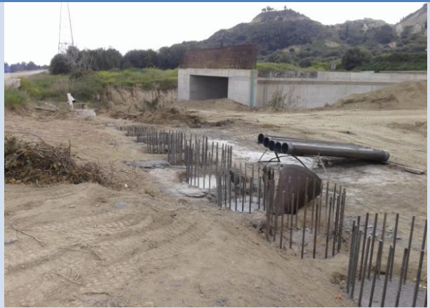
Retaining Structure G232: construction of piles
