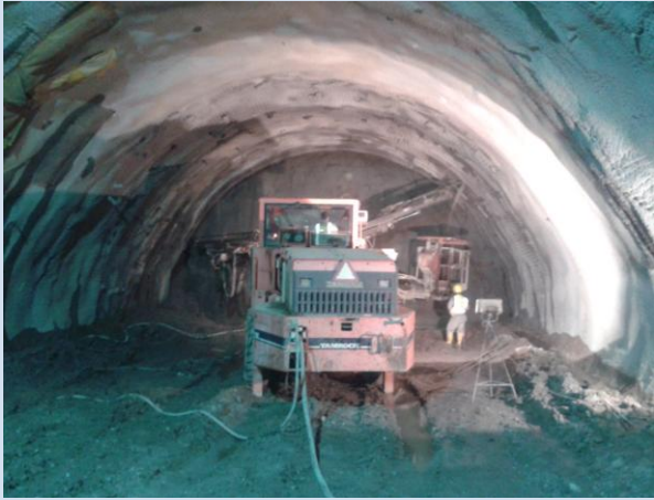
South Bore - A' Excavation Phase
