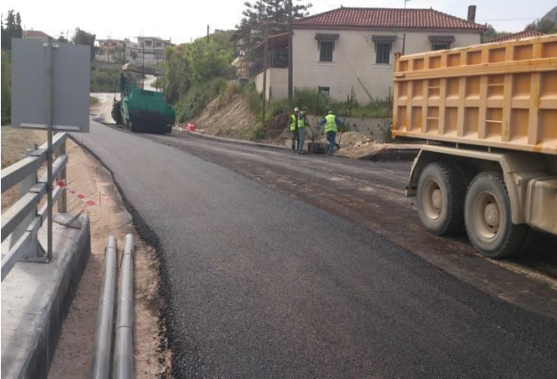
Asphalt works, A103
