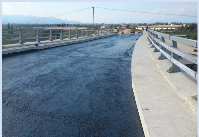
Waterproofing works, A103
