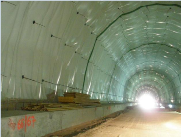
Mavra Litharia Final Lining-Waterproofing works
