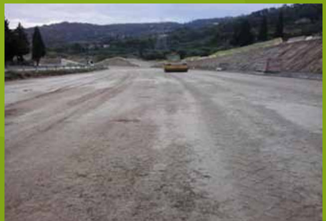
Earthworks-Ditches 22N-Derveni area
