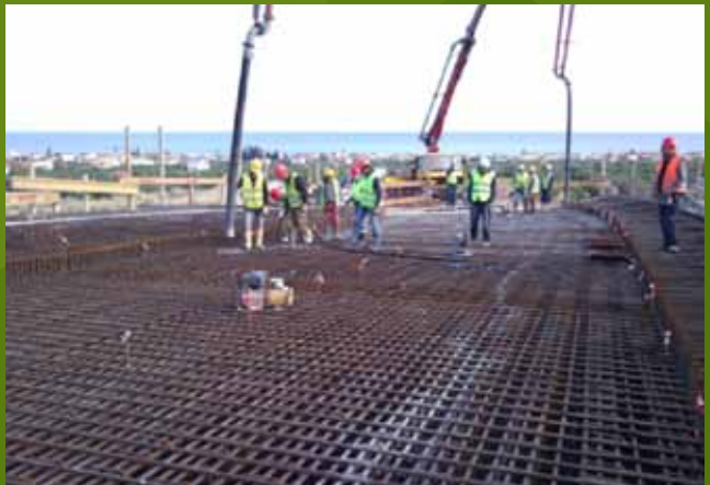
Overpass A223: Pouring deck slab
