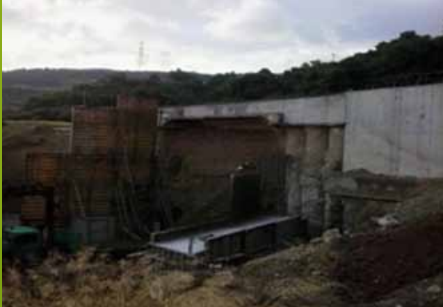
K247-Retaining Wall G.U. 23
