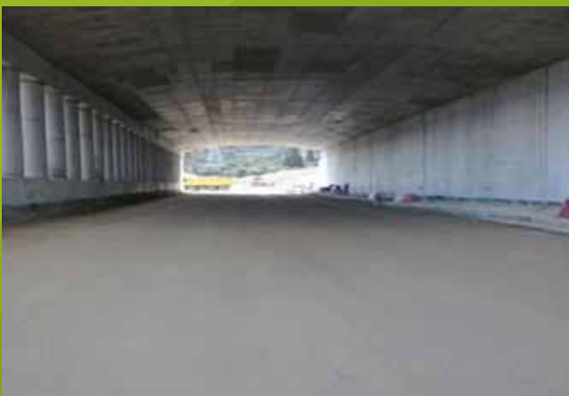
Lane Cover Derveniou – Pavement works
