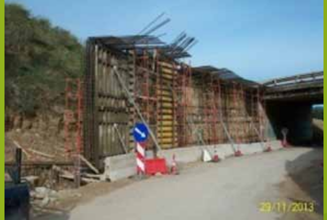
Ch 82+530 abutments pile construction at K282
