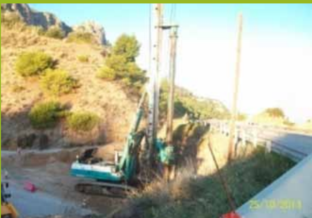
K270 ch 72+570 piles left branch
