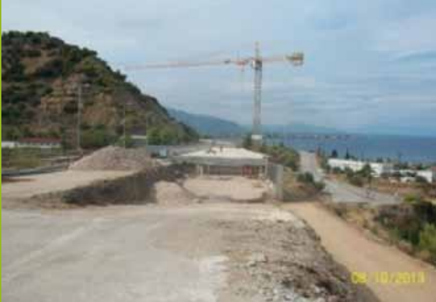
Ch 71+131 at B269 Ladopotamos- transitional embankment
