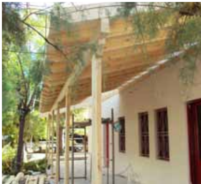
External ground roof – Storage House of 25th EBA
