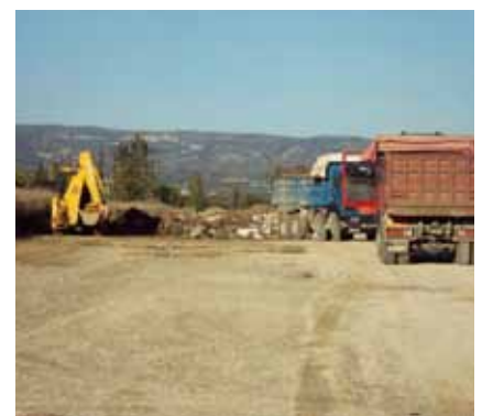
Cleaning of garbage at GU16 (k.p. 95+100)
