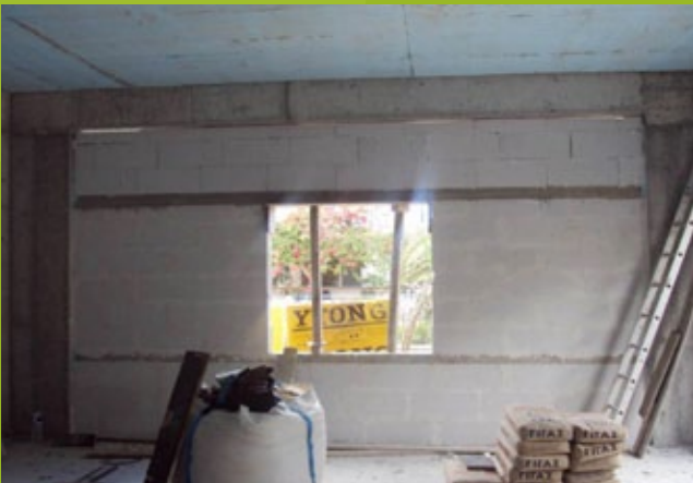
Exterior Masonry - ground floor - 25th EBA
