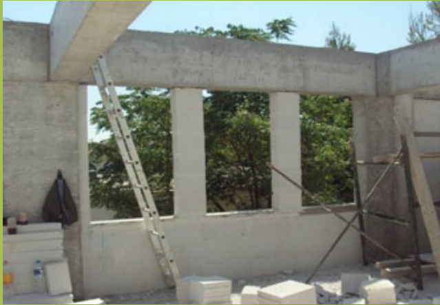
Exterior Masonry - 1st floor – 25th EBA
