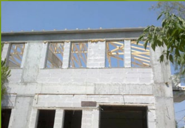
Roof Construction – 25th EBA
