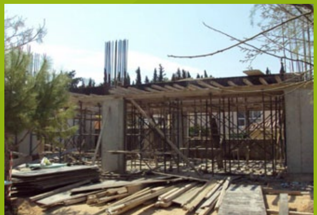
Ground floor upper slab – 25th EBA
