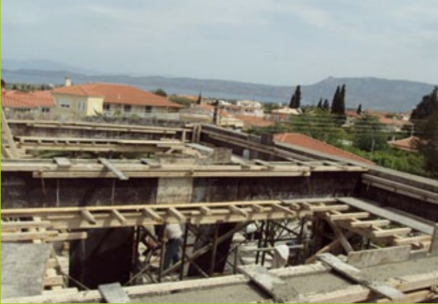
Concreting 1st floor columns and beams- 25th EBA
