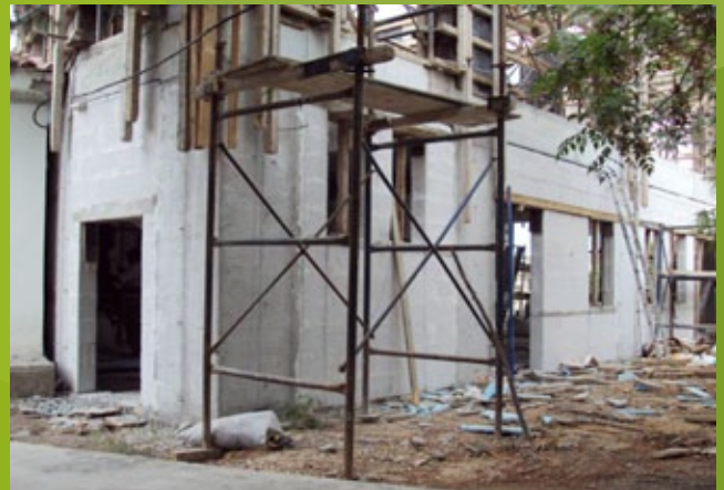
Exterior Masonry - ground floor - 25th EBA
