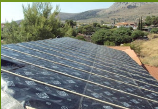
Roof Construction – 25th EBA
