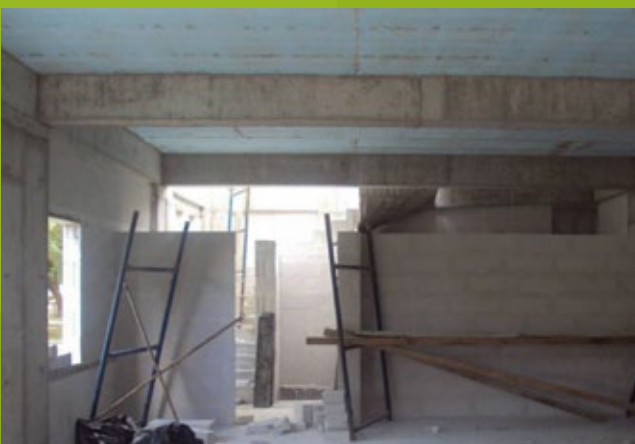
Interior Masonry - ground floor - 25th EBA
