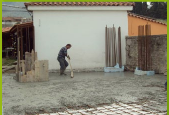
Ground slab – 25th EBA
