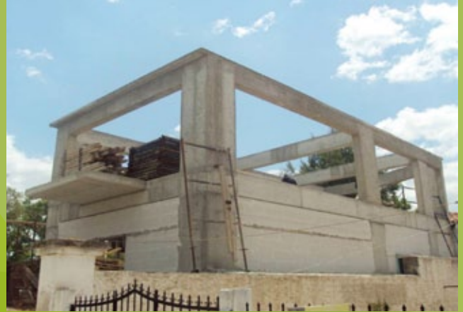
1st floor columns and beams- 25th EBA
