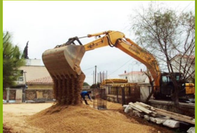
Foundation embankment – 25th EBA
