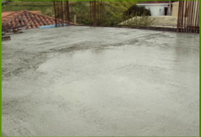
Concreting upper slab - ground floor – 25th EBA
