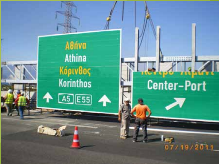
Horizontal signs installation
