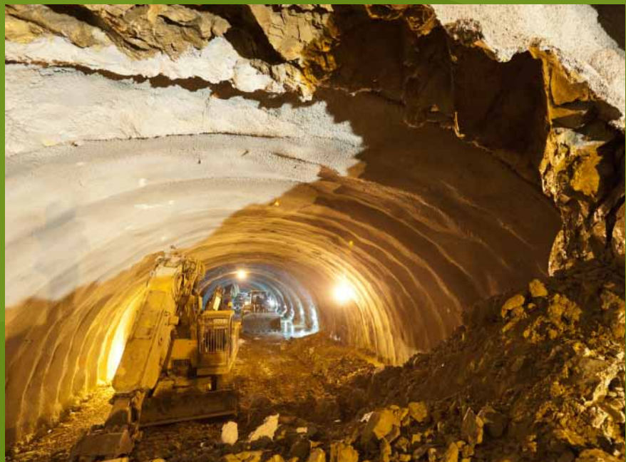
Tunnel 26 - excavation completion
