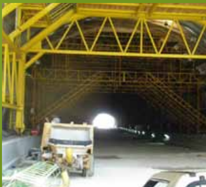
Tunnel 13B - Final lining works
