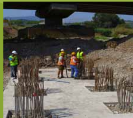
Meganitis River bridge construction works
