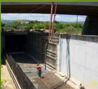
Bridge B131 (K.P. 19+320) - Structure 2nd Phase construction
