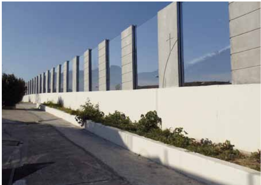
Installation of sound barriers, in the Project's existing sections (Zoodochos Pigi Abbey, Patra By-Pass)
