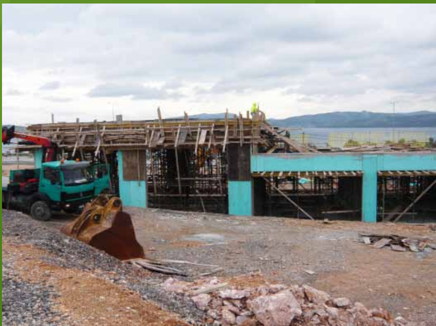
Concreting works for the MOMC in Nea Peramos
