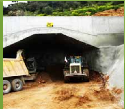
Tunnels A13 East Portal
