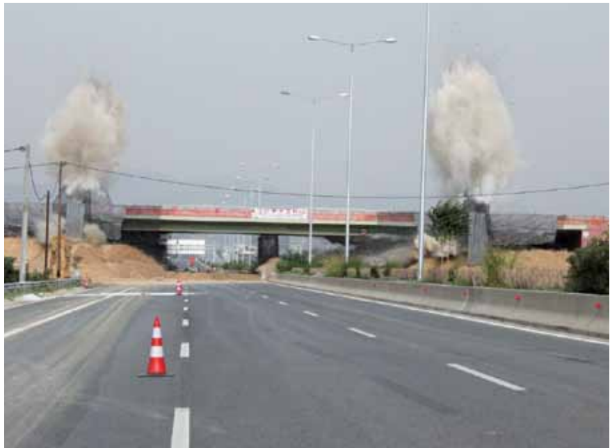
Vibration monitoring during Pachi bridge demolition
