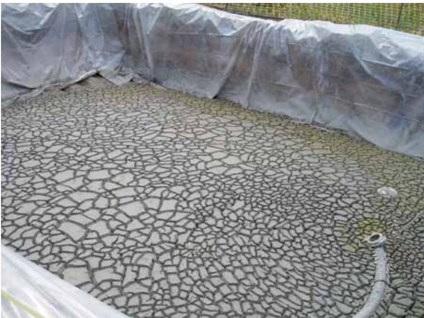
Bentonite reuse tank in Alfios River
