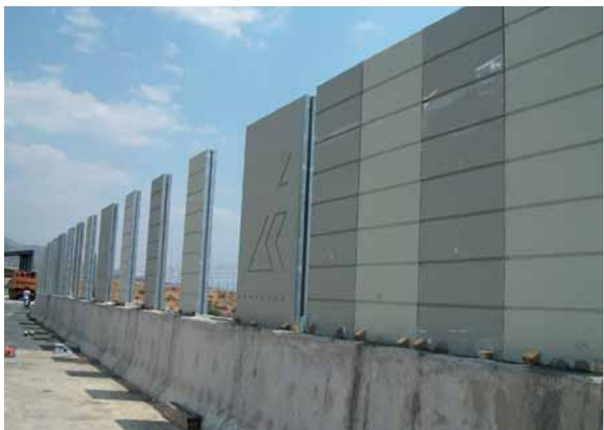
Sound barriers installation along Project's existing sections
