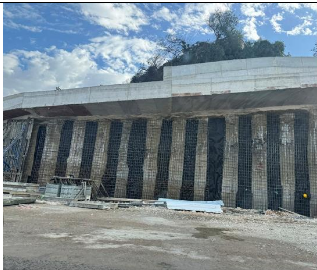
•Construction works for the Retaining Wall G670 (from k.p. 5+764,91 to k.p. 6+024,62)
