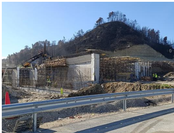
• Construction works for Underpass K710 (k.p. 6+948)
