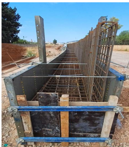
From k.p. 1+301 to k.p. 0+869 (right side): •Reinforcement/concreting works (pile cap, pile cap walls)
