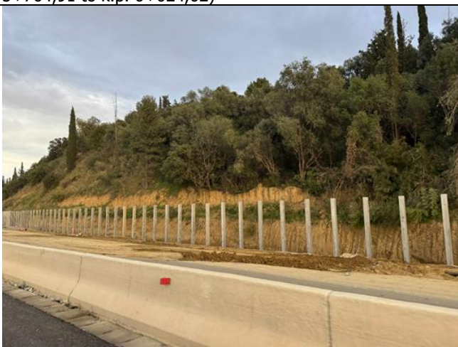
•Construction works for Retaining Wall G672 (from k.p. 0+633 to k.p. 1+001)
