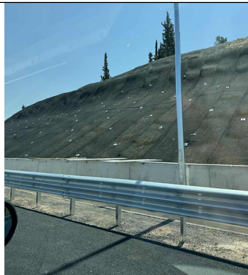
•Installation of nails and geogrid for the Retaining Wall G654 (from k.p. 9+070 to k.p. 9+295)
