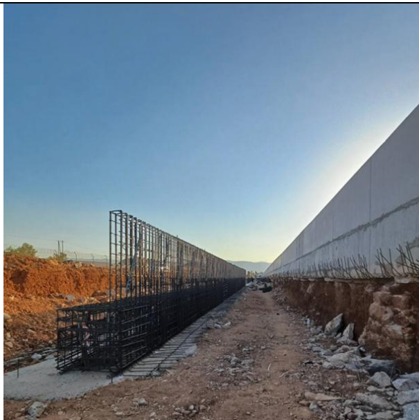
From k.p. 1+301 to k.p. 1+025: •Reinforcement/concreting works for pile cap
