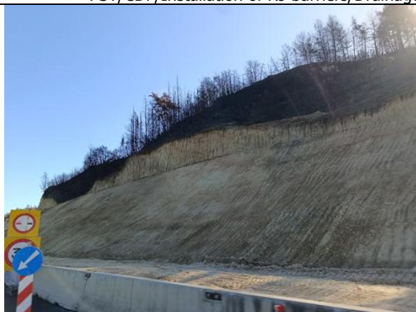
•Construction works for VIPE Interchange (k.p. 6+950)
