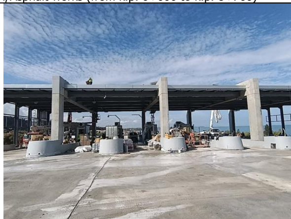
•Surrounding area/rigid pavement/E-M installations works at Frontal Toll Station (k.p. 8+450)
