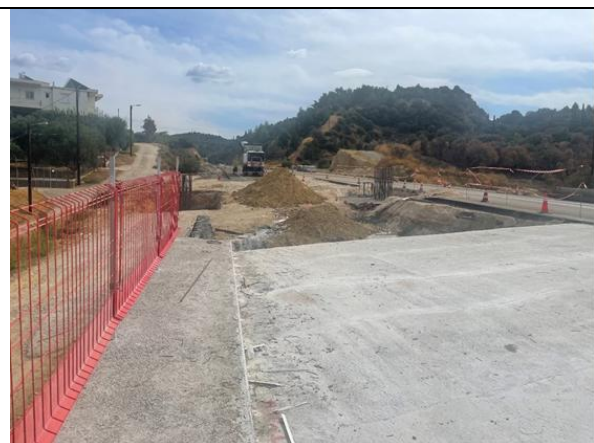
•Construction works for Underpass K706 (k.p.4+057,23)
