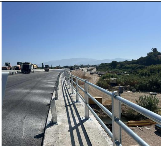
•Waterproofing/Asphalt/Installation of safety barriers/installation of handrails works for the Bridge B801 (k.p. 12+916,00)
