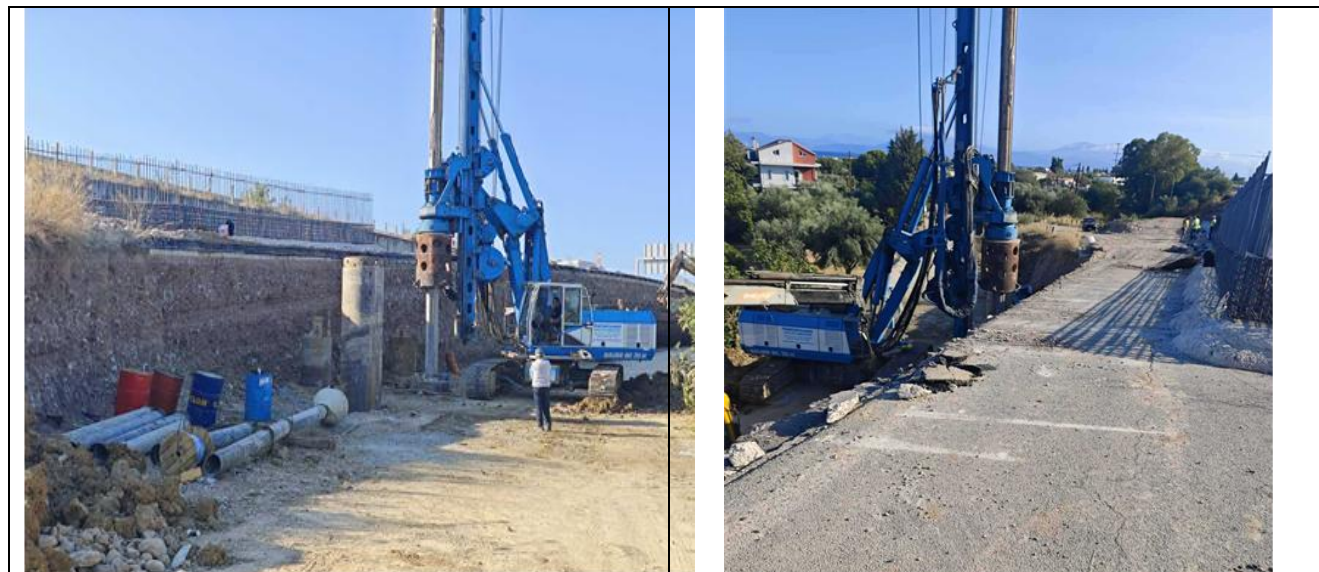
Construction works for the Retaining Walls R01, R02, R03 at Midilogli semi-interchange (k.p. 0-001,95)
