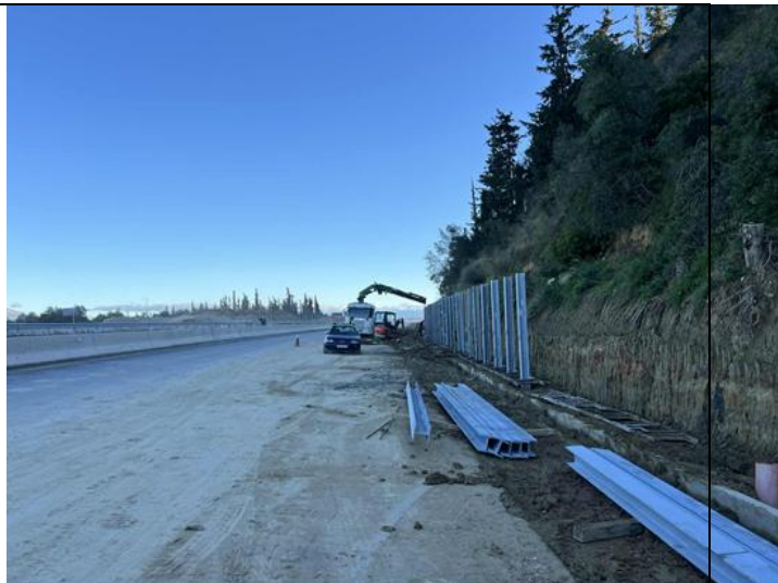
•Construction works for the Retaining Wall G672 (from k.p. 0+633 to k.p. 1+001)
