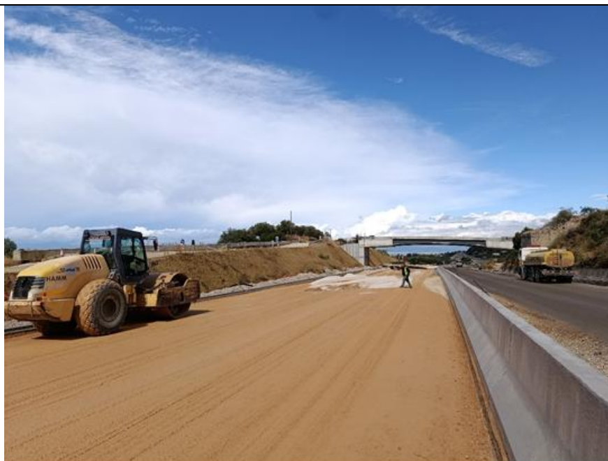
•PST/CDF/Installation of NJ barriers/Drainage/E-M/Asphalt works (from k.p. 0+000 to k.p. 8+700)
