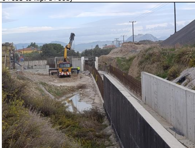
•Construction works for Box Culvert L631 (k.p. 6+925,64)
