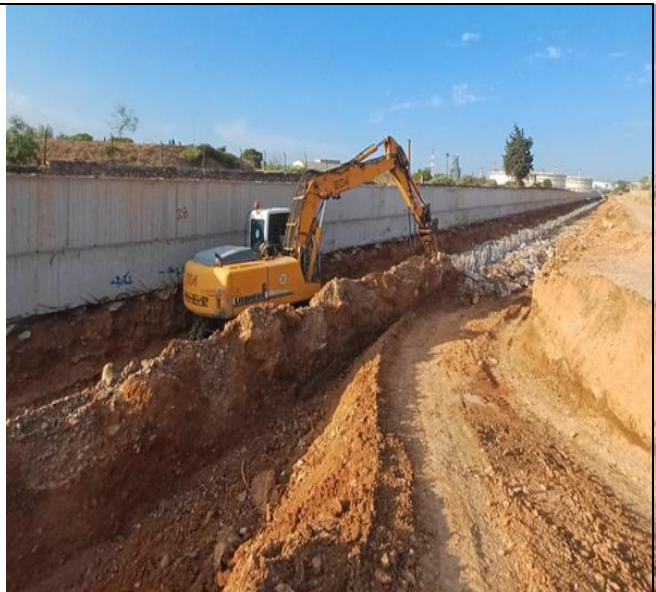
From k.p. 1+301 to k.p. 0+850: •Cleaning works for pile cap
