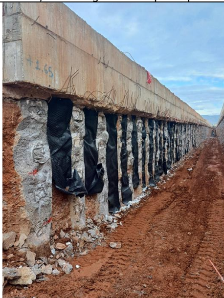
From k.p. 1+301,05 to k.p. 1+250: •Drainage membrane installation works (walls between piles)
