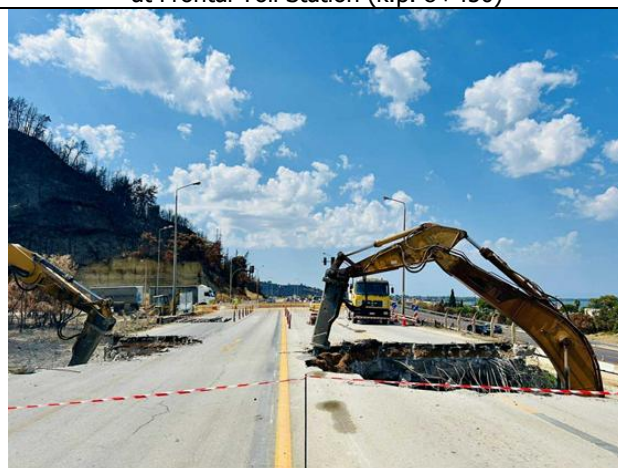
•Demolition of existing wall/construction works for the Underpass K710 (k.p. 6+948)
