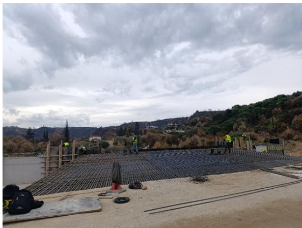
•Construction works for Underpass K705 (k.p. 3+469,84)
