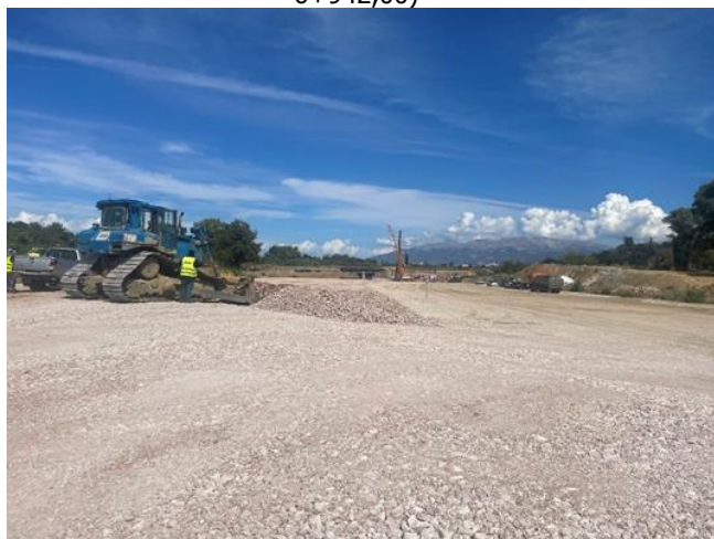
Construction works for the Underpass K703 (k.p. 1+980)
