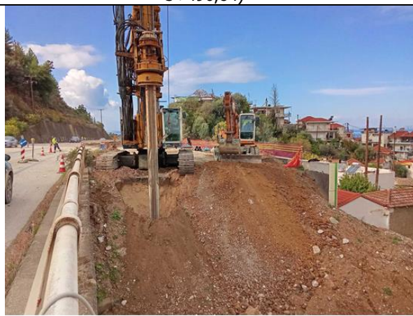
Construction works for the Retaining Walls G665 (from k.p.
