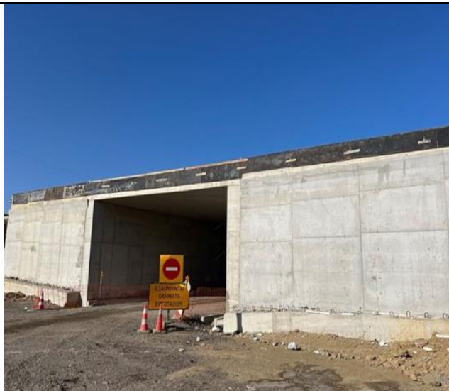
Construction works for the Underpass K708 (k.p. 6+098,46)
