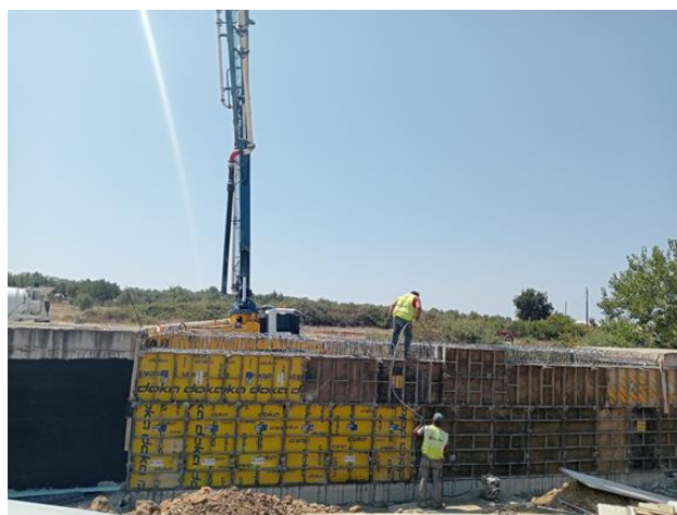
Construction works for the Bridge B801 (k.p. 12+916)
