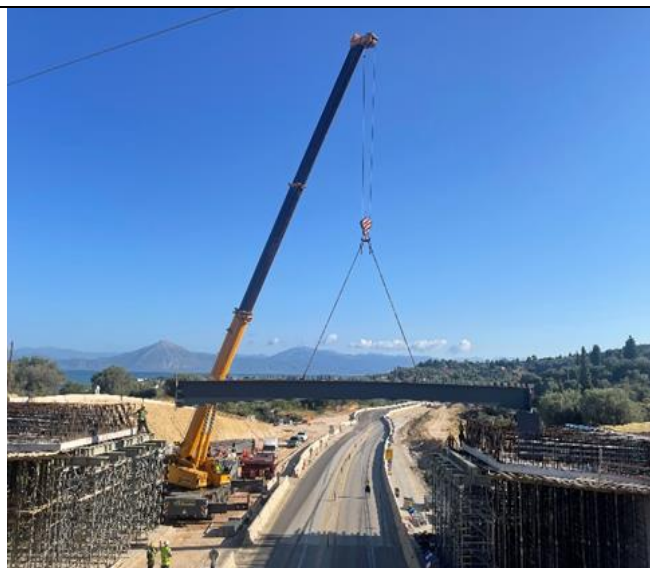
Construction works for Box Culvert L620 (k.p. 3+295)
