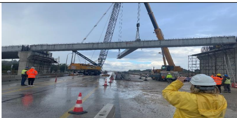
Construction works for Overpass A714, k.p. 11+733,41
