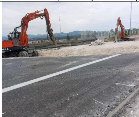
Existing Structure K037: Demolition works for the upper slab of the structure (section 2)
