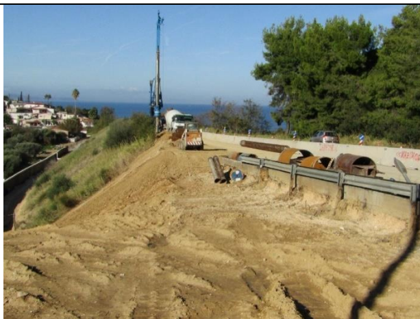
Construction works for Underpass K706, k.p. 4+057.23
