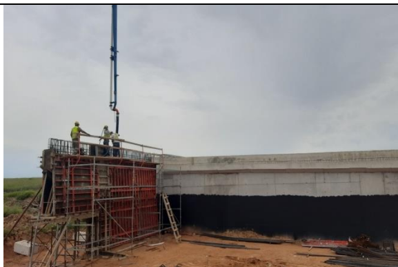
K819 (k.p. 40+279): Reinforcement/Formwork/Concreting
