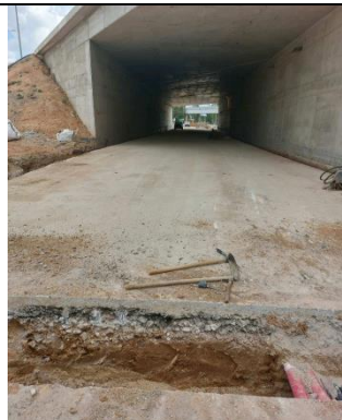
Existing Structure K007: E/M works (central island)
