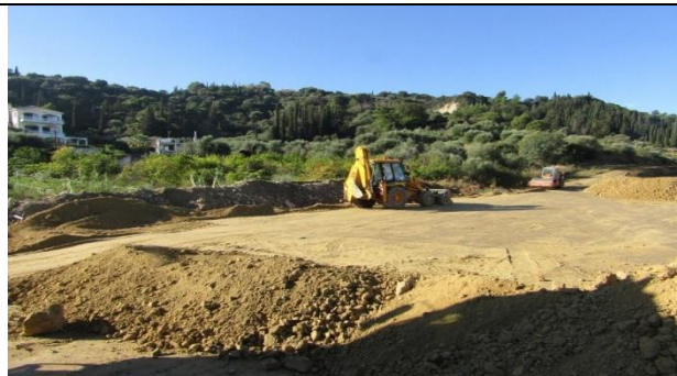
Construction works K708, k.p. 6+098,46
