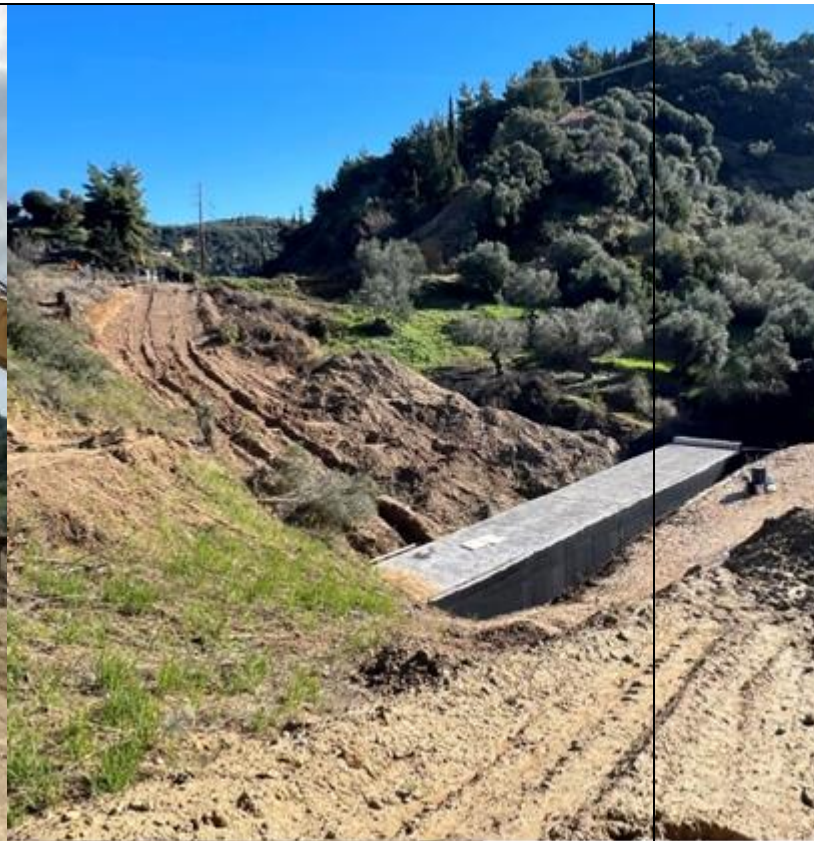
Construction works for Box Culvert L622, k.p. 3+875,81
