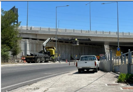
Existing structure K603: Installation of deck drainage pipe
