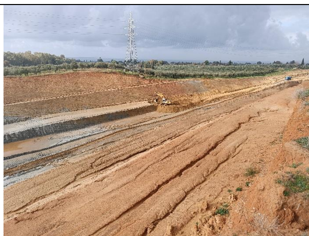
Excavation works Gastouni-Pyrgos
