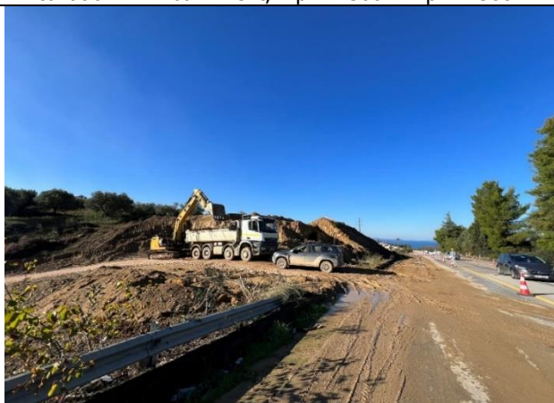
Excavation works, k.p. 3+900
