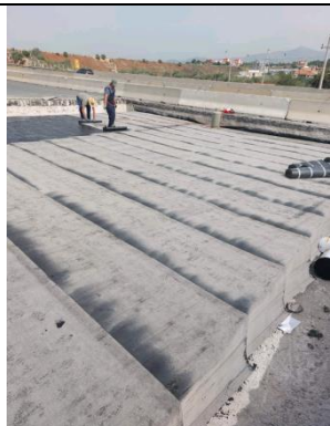
Existing Structure K013: Completion of rehabilitation works (phase 3 – left branch)
