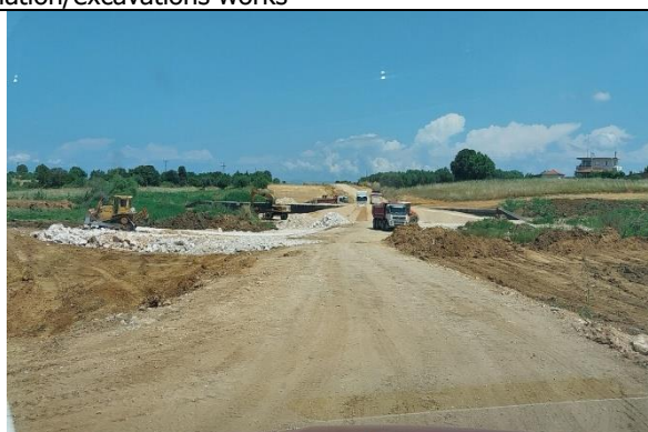
L808 (k.p. 39+000): Top soil removal and soil improvement works
