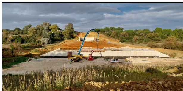
concreting (B816), k.p. 42+130
