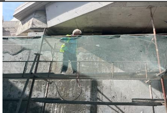
Existing structure K603: Restoration of the abutments' surfaces
