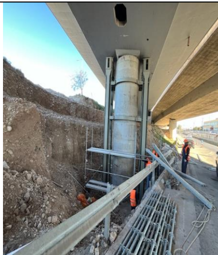
Existing structure B601: Installation of the base metal structure for the lifting jacks for (M1)
