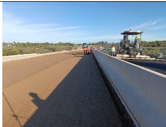
Construction of CDF Gastouni-Pyrgos
