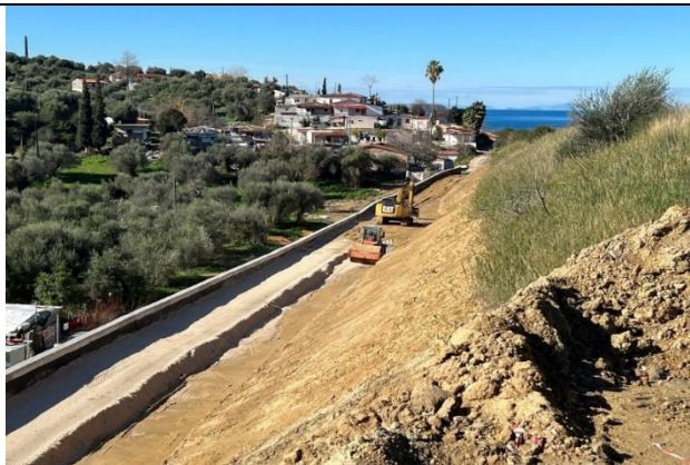
Construction works for Retaining Wall R610, k.p. 4+064,90 – k.p. 4+266.05
