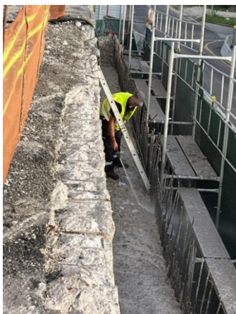
Existing structure K603 Demolition works for the upper part of the bearing area of the existing abutments
