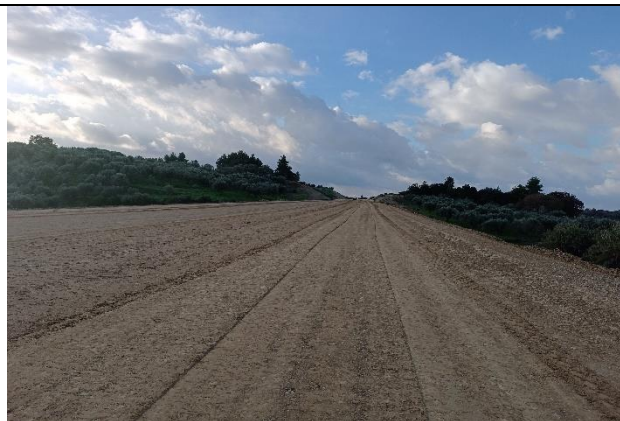
Construction of PST Gastouni-Pyrgos
