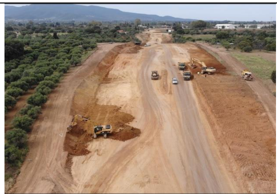
Excavation works - embankment (k.p. 14+000 – k.p. 14+500)
