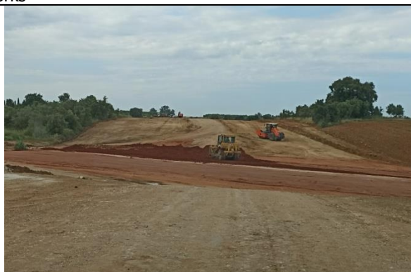
L811 (k.p. 39+970): Top soil removal and soil improvement works
