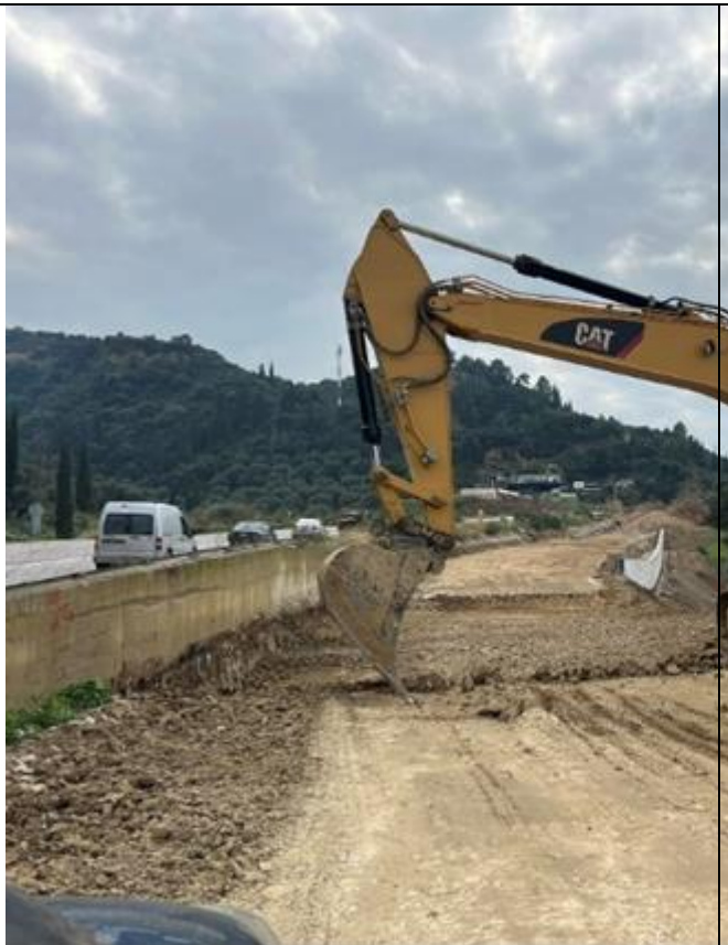
Excavation – Embankment, k.p. 2+300 – k.p. 2+500
