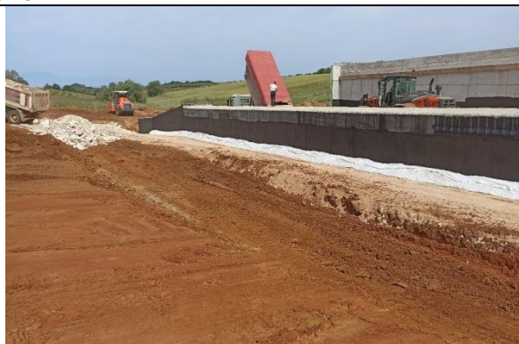
L812 (k.p. 40+297): Soil improvement works, Side drain
