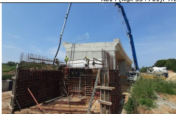
A816 (k.p.34+822): Concreting works
