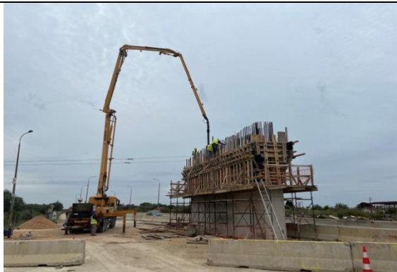
Construction works for Overpass A714, A715 (k.p. 11+733,41)
