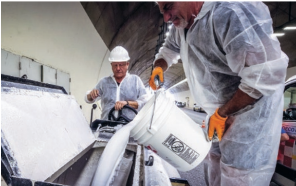
2. Mixing of the components of the coating
