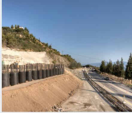
The two typical types of retaining structures found on Olympia Odos is the "lane cover" and the "pile wall". The use of such type of retaining structures enables us to minimize our intervention in the geomorphological environment. We "drive" the road through such structures instead of cutting the mountain on 20-30 meters. This is a slightly invasive method compared to the practices used in the past.
