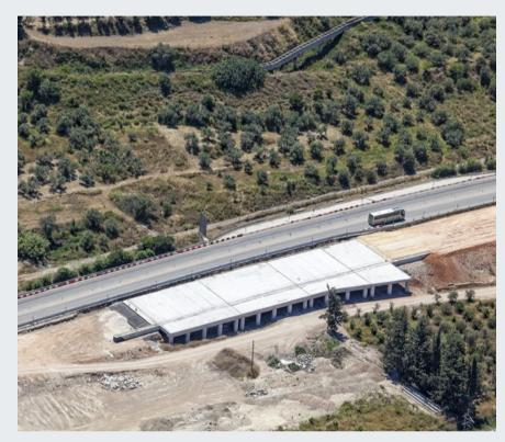
The archaic wall of Corinth (very close to the Justinian Wall) is beneath this particular structure. To protect and make this particular find accessible, the most appropriate solution was to construct a bridge instead of the so-called "embankment technique". In fact we constructed a bridge in order to divert the traffic over this find without putting at risk the antiquities.
