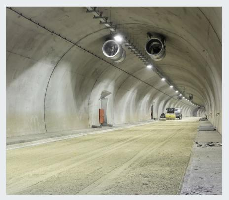
Regarding the tunnels we construct at Derveni, Akrata, Panagopoula and Platanos, we use the so-called "New Austrian Tunneling Method" (NATM), i.e. conventional means using machinery and excavation steps, instead of the well-known Tunnel Boring Machine constructed for specific cross-sections and highly expensive. See views of Panagopoula tunnels, one of which is a 4km twin bore tunnel (two traffic directions).
