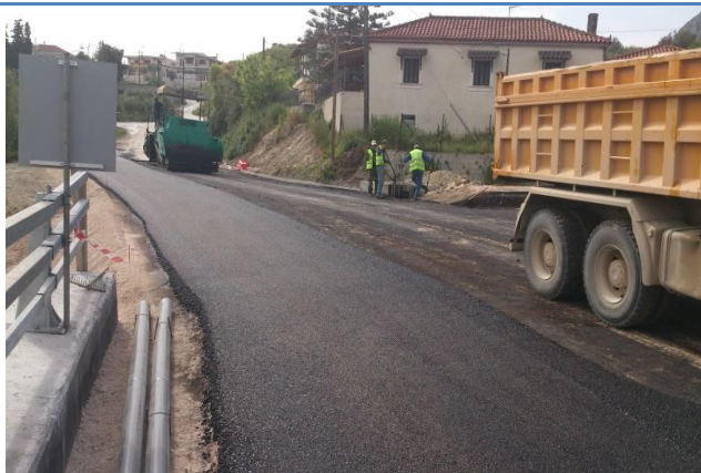
Asphalt works, A103
