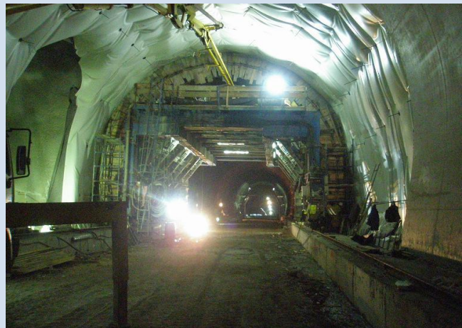
Mavra Litharia Final Lining-Concrete works
