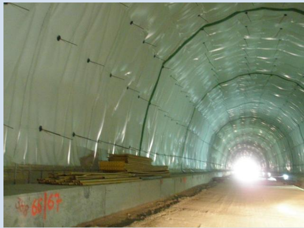
Mavra Litharia Final Lining-Waterproofing works
