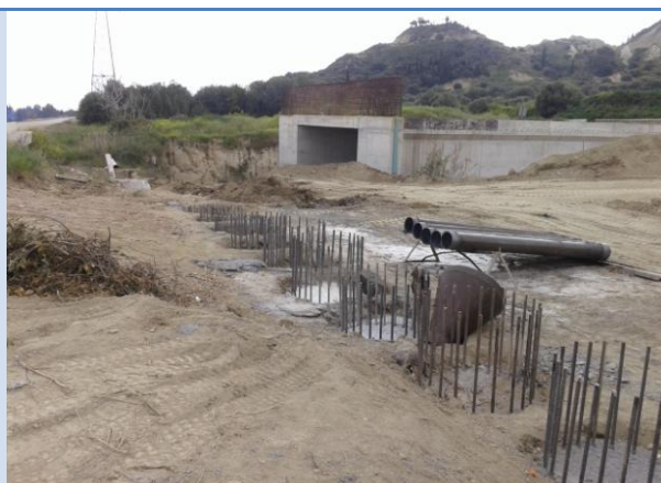
Retaining Structure G232: construction of piles
