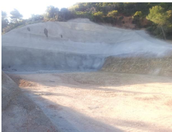
T25_west portal cover & cut open excavation
