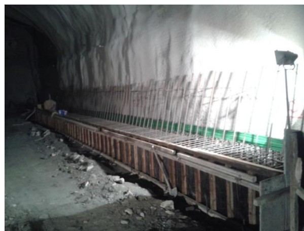
Implementation of final lining - (Footing) Cross Passage 2
