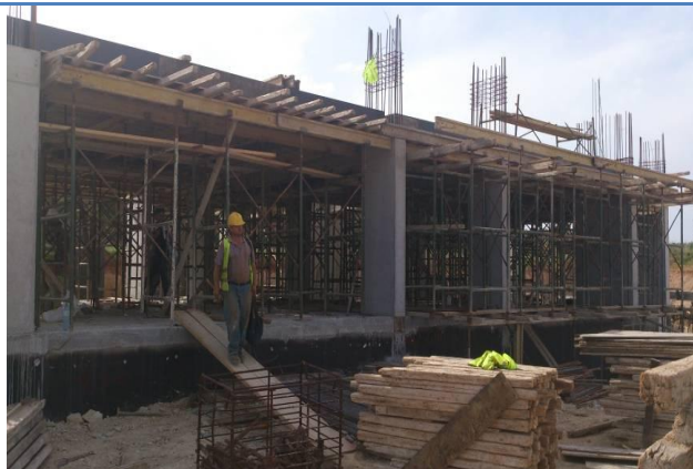
Construction of TAB, k.p. 18+800
