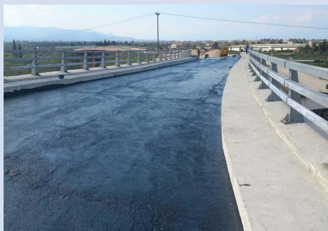
Waterproofing works, A103
