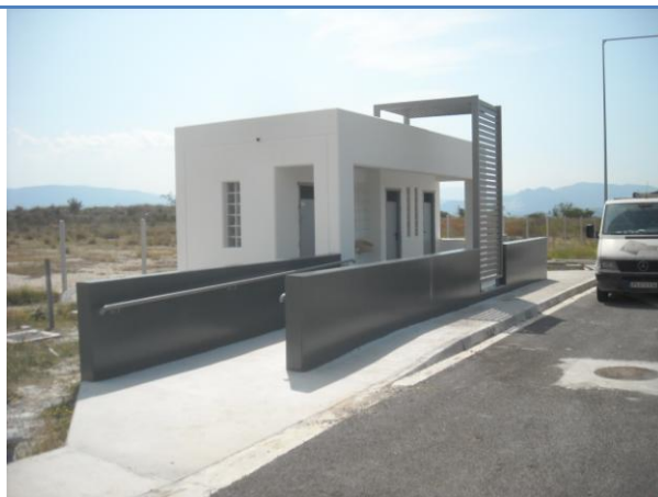
Kalamaki parking area direction to Elefsina – Finishing works
