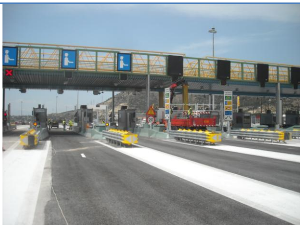
Isthmos Toll Station
