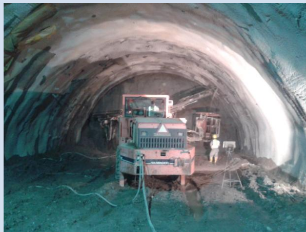
South Bore - A' Excavation Phase
