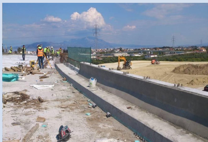
Construction of top slab, A137
