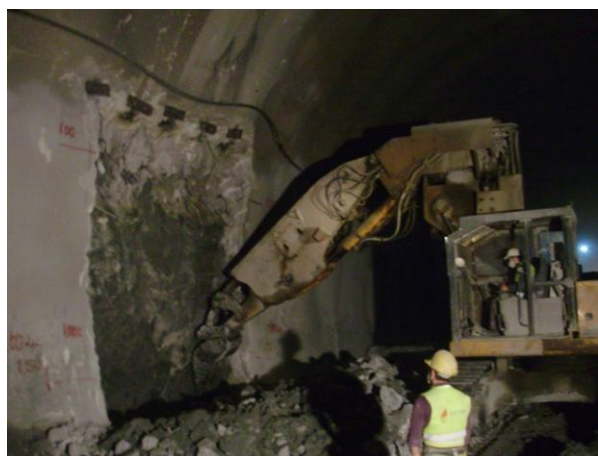
South Bore - B' & C' Excavation Phase
