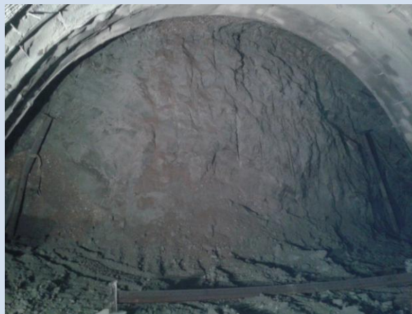
North Bore - A' Excavation Phase
