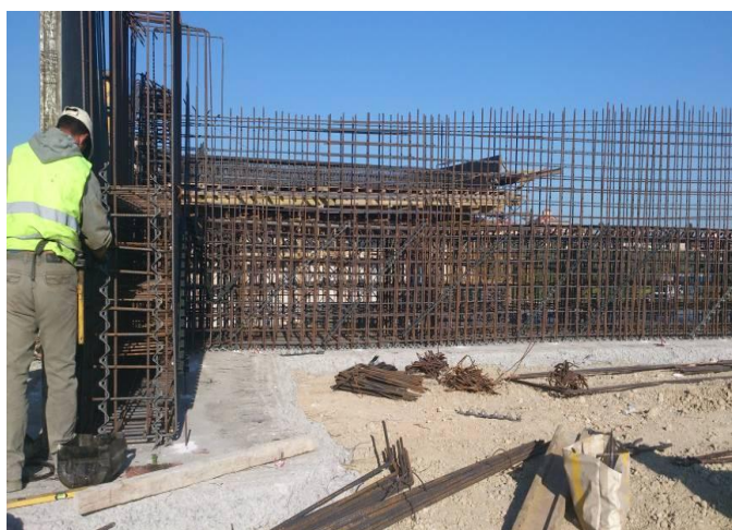
Construction of Abutment A0, A137
