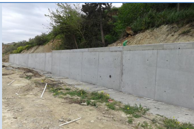
Retaining Structure G247
