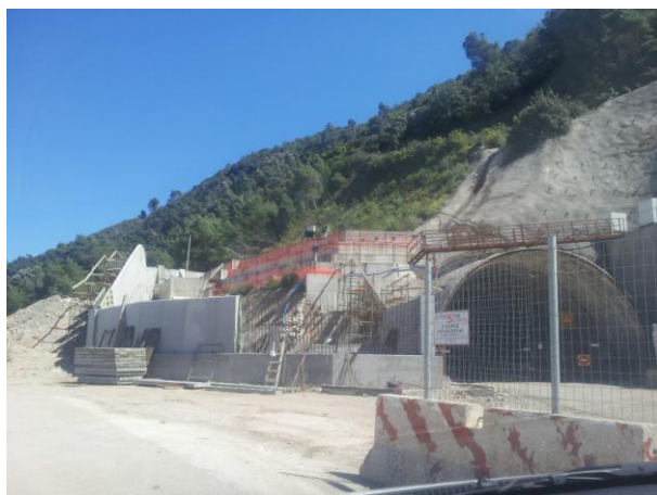
T26_NW retaining walls
