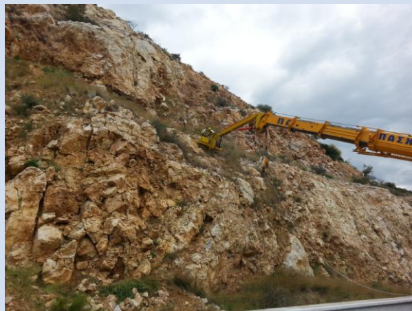
Loose rock removal
