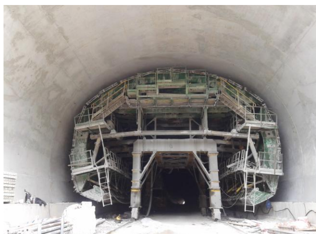
Cut & Cover T007 West: segment 2
