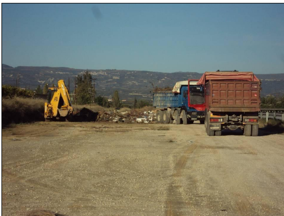
Cleaning of garbage at GU16 (k.p. 95+100)
